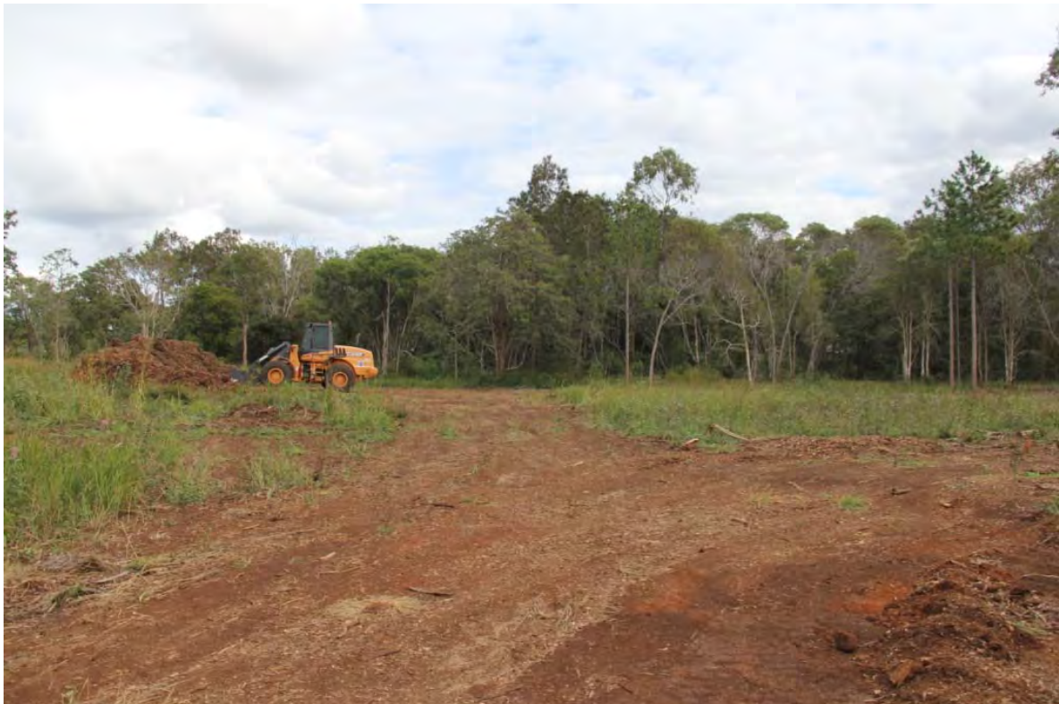
Figure 6 - Low Value Rehabilitation area looking south
