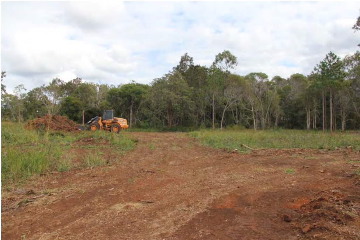
Figure 6 - Low Value Rehabilitation area looking south
