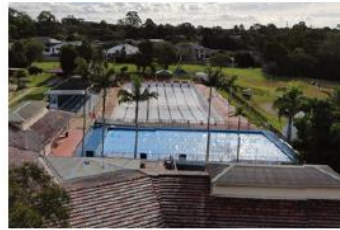
Cleveland Aquatic Centre upgrades
