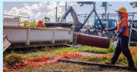
School of Arts Road sewer upgrade
