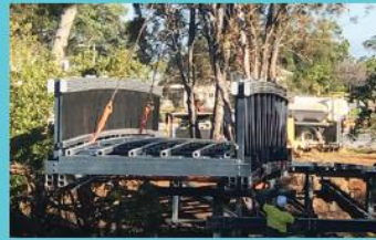
Weinam Creek footbridge installation
