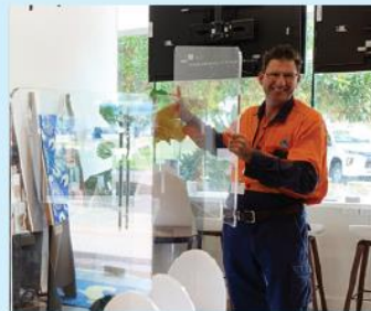
Perspex screens being installed
