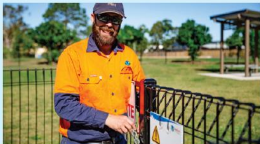
Safety signage being installed
