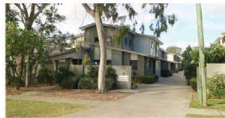
Figure 1: The access road has been positioned to the west of the buildings so that the private side alfresco/courtyards and living spaces for the units can benefit from natural light and ventilation from the north and east.
