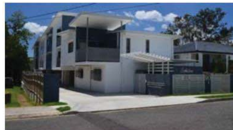
Refuse storage located within the site and with screening and good ventilation.
