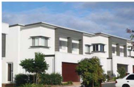
Variation in building depth, hoods, projections and screening provides solar access and effective shading.
