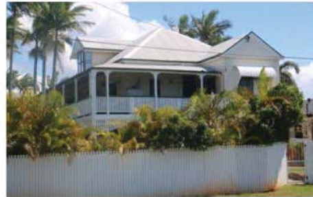
Addresses both street frontages Multiple roof pitches and varying heights Projections and recesses in façade Outdoor living – wrap around covered balcony
