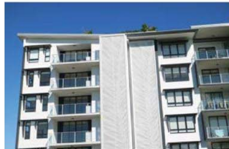
This apartment block has a north eastern aspect. The artistic screening provides a distinct identity and gives vertical emphasis to break up the long façade.
