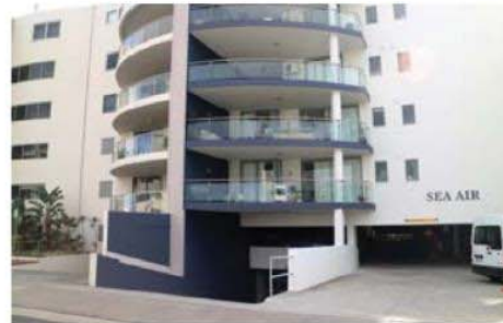
For apartments, the impact of vehicle access points can be minimised by locating them on secondary/rear frontages.
