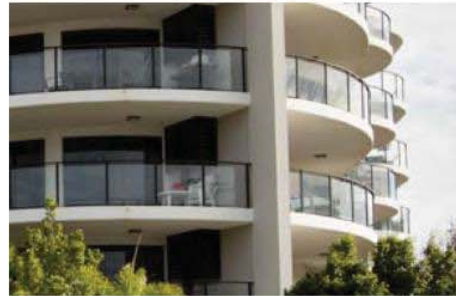
Balconies enhance the amenity and indoor/outdoor lifestyle of residents. Building articulation such as balconies and deeper window-reveals provide visual interest to the façade.
