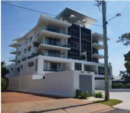
Services and plant need to be easily accessible for maintenance but can be designed to blend in with overall design and simple palette
