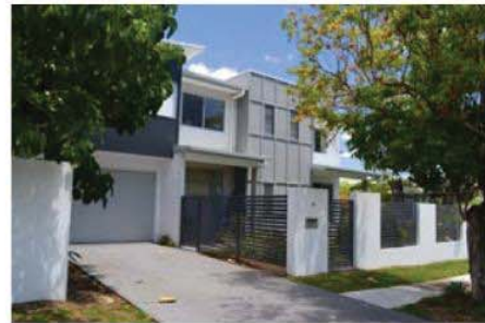
Fencing materials allow for casual surveillance whilst also maintaining privacy for residents.
