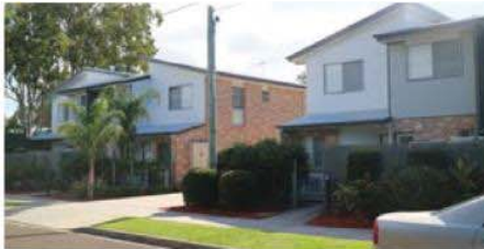
Figure 4: Varied depth of façade and articulation of roof line together with the cohesive palette of brick, render and light weight cladding creates an interesting streetscape.
