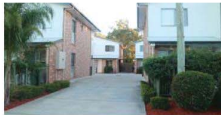
Figure 6: Parking, bin storage and services are discretely located behind the building to improve the visual appearance of the development from the street.
