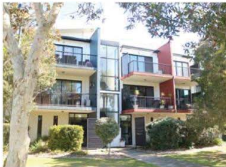
Common corridors and stairwell designed to be naturally lit.
