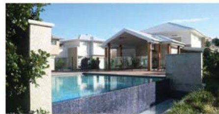
Figure 9: Communal open space offers privacy but also benefits from passive surveillance. There are three areas of communal space in this development to cater for differing settings.
