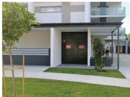
Services and plant discreetly housed near mail boxes.
