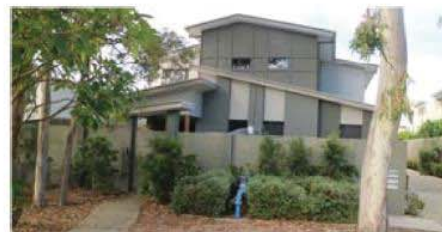
Figure 2: Building façade articulation, varied skillion roof form and mixed material fencing provide interest to the street. The complementary material and colour palette of the built structures are softened by vegetated landscaping. The street interface could be improved by lower fencing, or increased transparency in the fencing.
