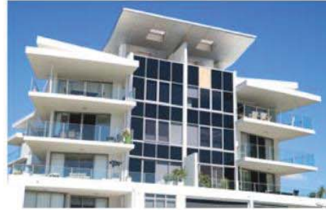
Dual aspects apartments with doors and windows that can be opened maximise natural ventilation opportunities. Common lift areas have natural light.
