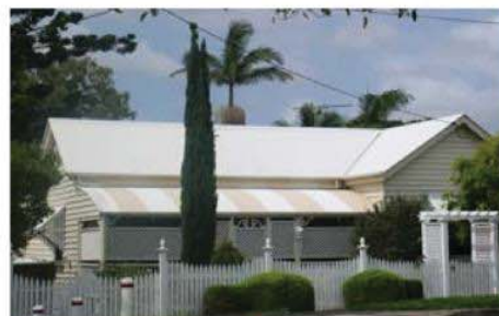
Bull nose roof on verandah Timber picket fence Light with materials, timber frame and corrugated iron Articulated entrance with timber arbour Landscape strip along frontage
