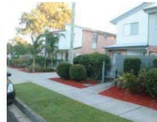
Units address the street with direct pedestrian access which balances openness with privacy.
