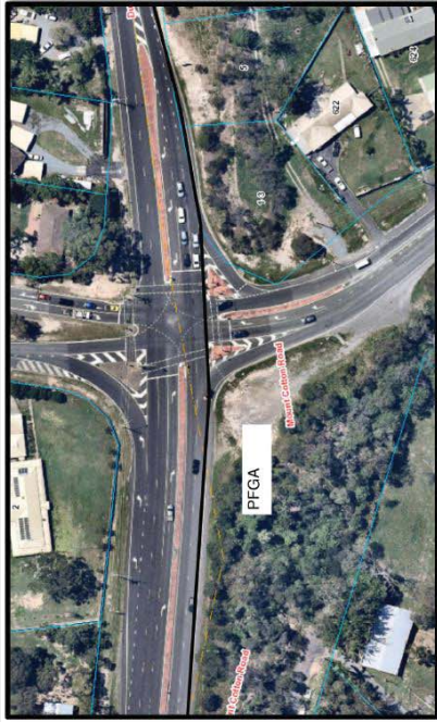
Figure 27 – Boundary Road and Mt Cotton Road intersection
