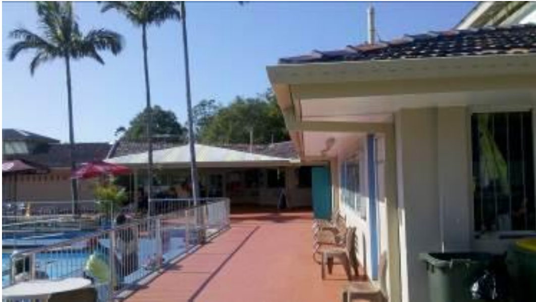
Image 12 Cleveland Aquatic Centre 25m Pool Concourse
