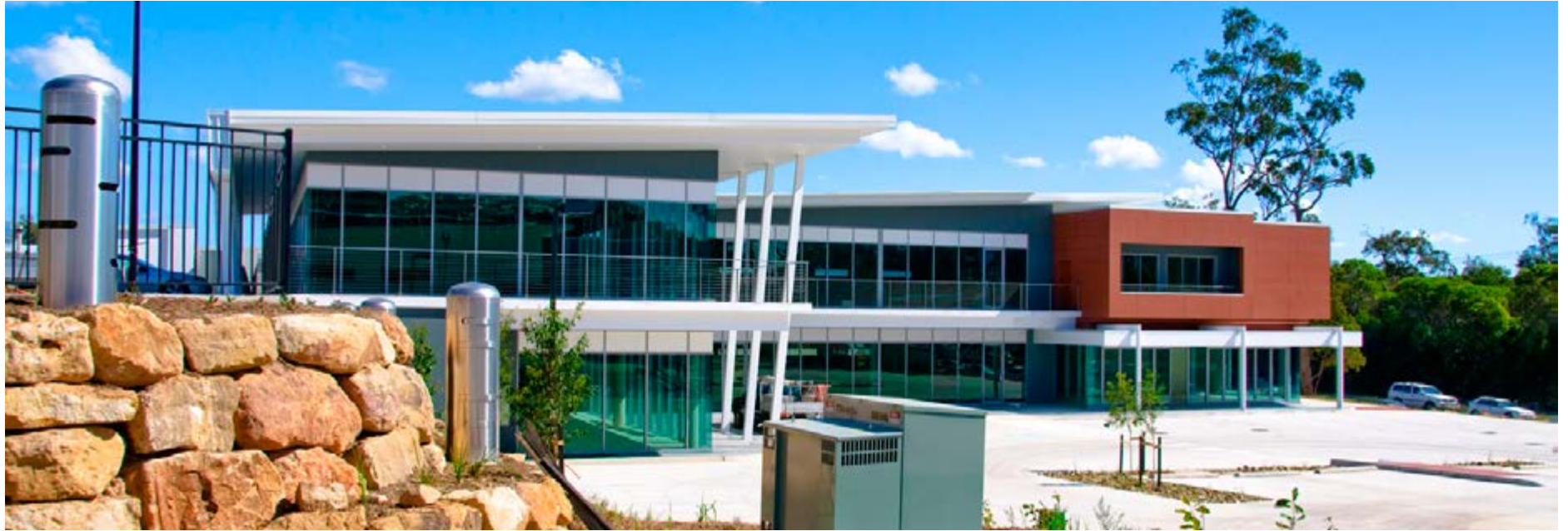
Business complex at Cleveland
