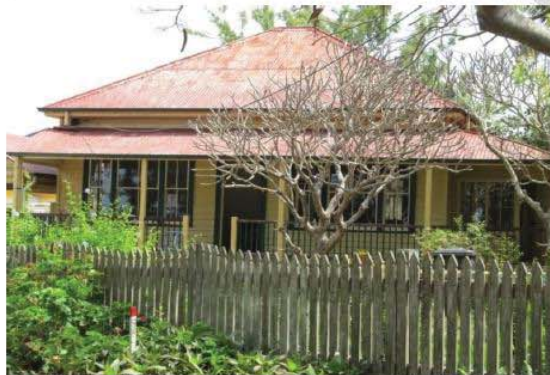
Residence, 17-18 The Esplanade, Wellington Point (RCC, 2012).
