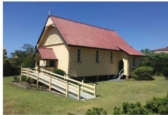
St James' Anglican Church, Wellington Point (AHS, 2016).
