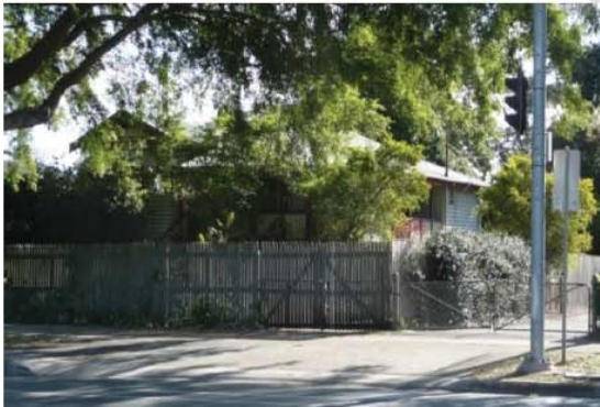
Wellington Point School Principal's House (Former), Wellington Point (AHS, 2016).
