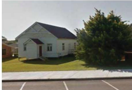
Methodist Church Hall, Cleveland (AHS, 2017).
