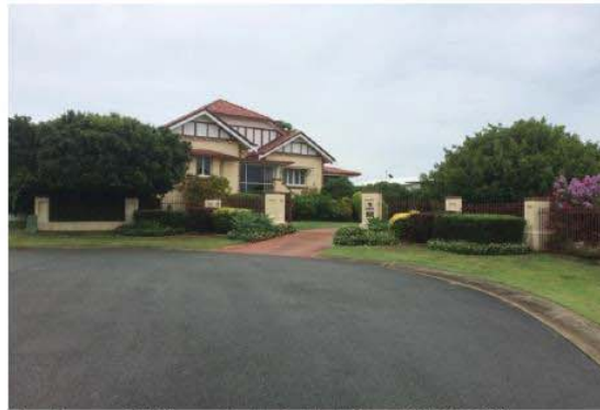
Residence, 6 Melrose Court, Redland Bay (AHS, 2016).
