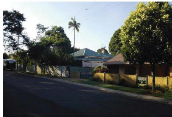
Residence, 6 Harris Street (AHS, 2016).
