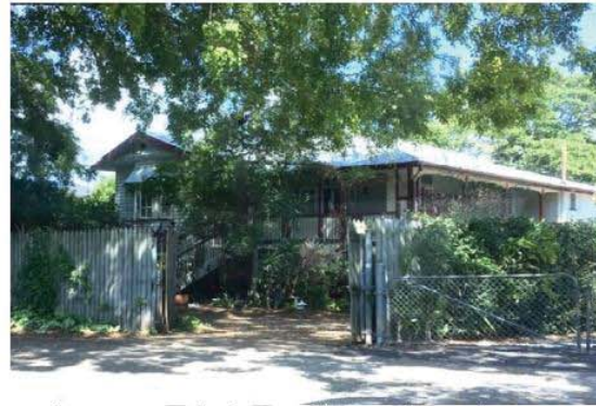
Wellington Point School Principal's House (Former), 480-482 Main Road (AHS, 2017).
