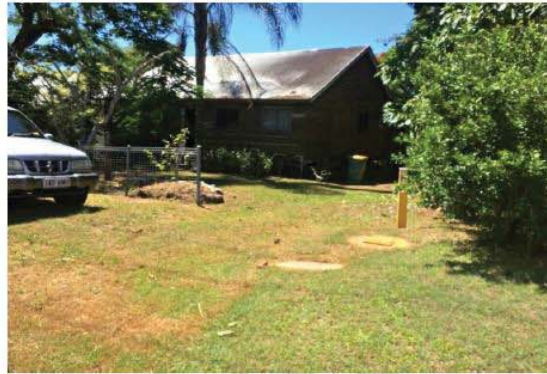
Residence, 11 Parsons Street, Dunwich (AHS, 2016).
