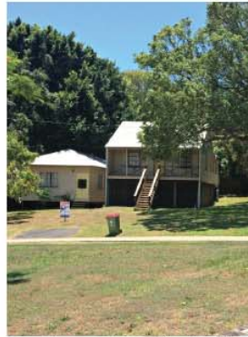
Residence, 12 Stradbroke Place, Dunwich (AHS, 2016).
