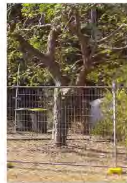
TREE PROTECTION FENCE No.1 TPF1 - 1800 high steel mesh fence. Installed following survey setout fence to be supported on, clamped and to have Arborist signage cable tied fixed in place.
