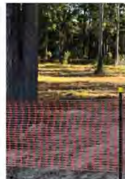
TREE PROTECTION FENCE No.2 TPF2 - Orange mesh with steel staking to be used in support locations and where ground conditions limit the access for TPF1. Fence line to be based on surveyed positioning.
