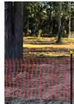
TREE PROTECTION FENCE No.2 TPF2 - Orange mesh with steel staking to be used in support locations and where ground conditions limit the access for TP1. Fence line to be based on surveyed positioning.
