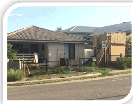
Photo 1: Children's play fort visible from non-access street – Grande Ave, Springfield Lakes.
