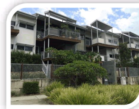
Photo 6: Example of two storey dwellings with balconies overlooking non-access street
