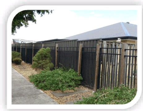
Photo 3: Installation of colorbond fencing internal to semi-transparent fencing to achieve privacy
