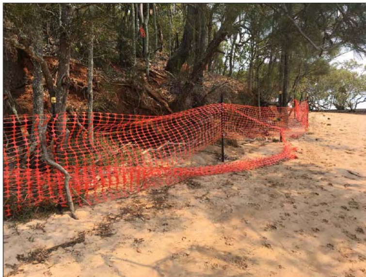
Figure 4.3 Eroding bank, Wellington Point foreshore.
