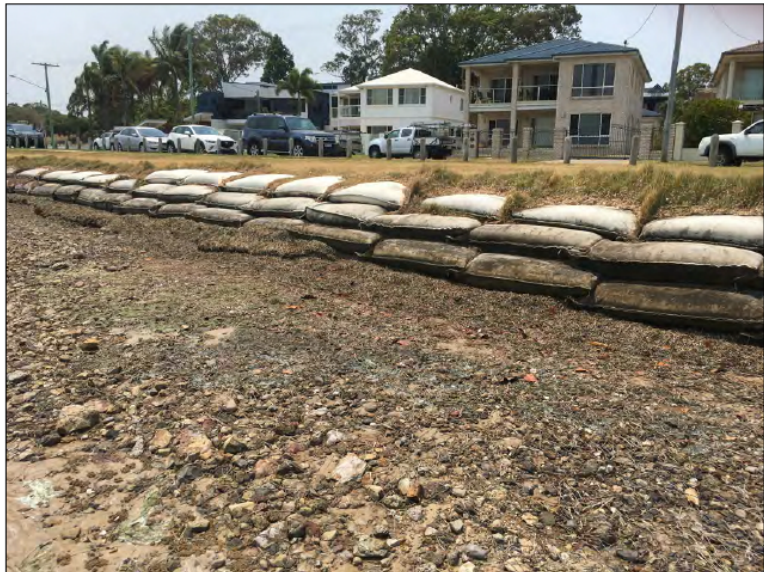
Figure 3.4 Sandbags along the foreshore Queens Esplanade, Thorneside.
