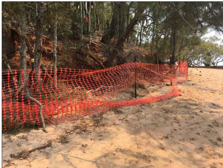
Figure 4.3 Eroding bank, Wellington Point foreshore.
