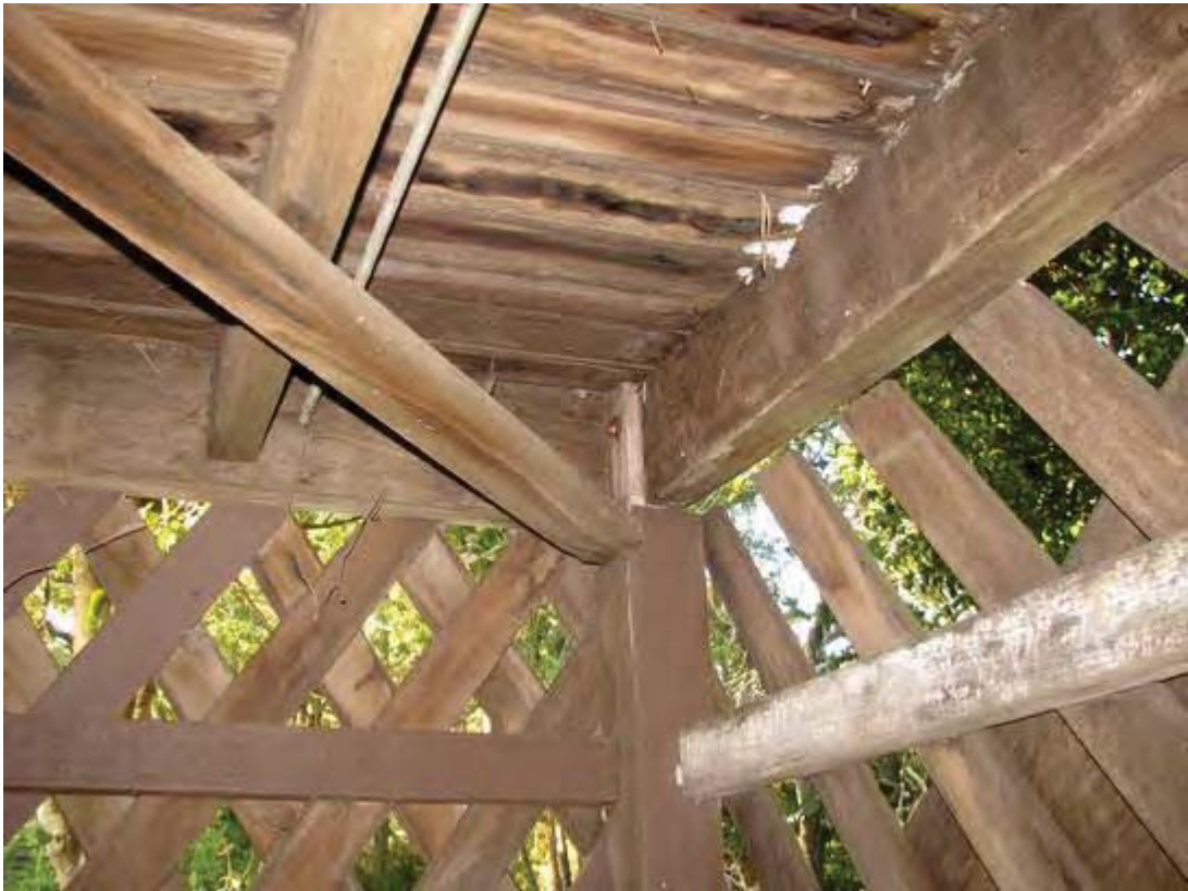
Photograph 9 - Residence verandah subfloor
