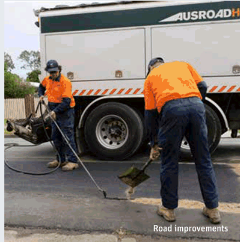
Sensors in use
