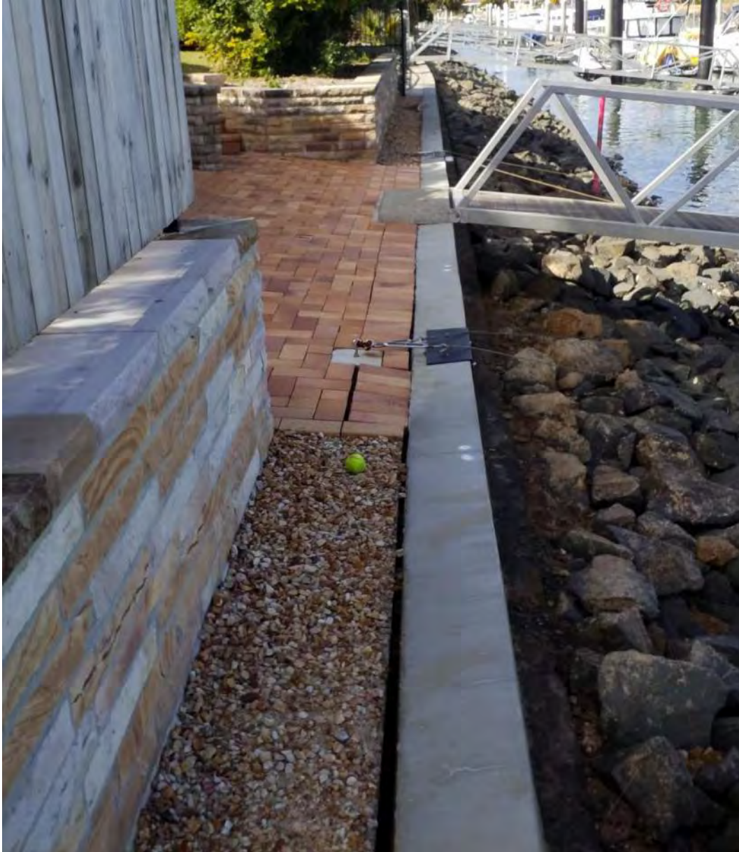
Figure 36: 81 Masthead Drive - Post-construction general view looking east, dated 20 June 2018 (from [12])
