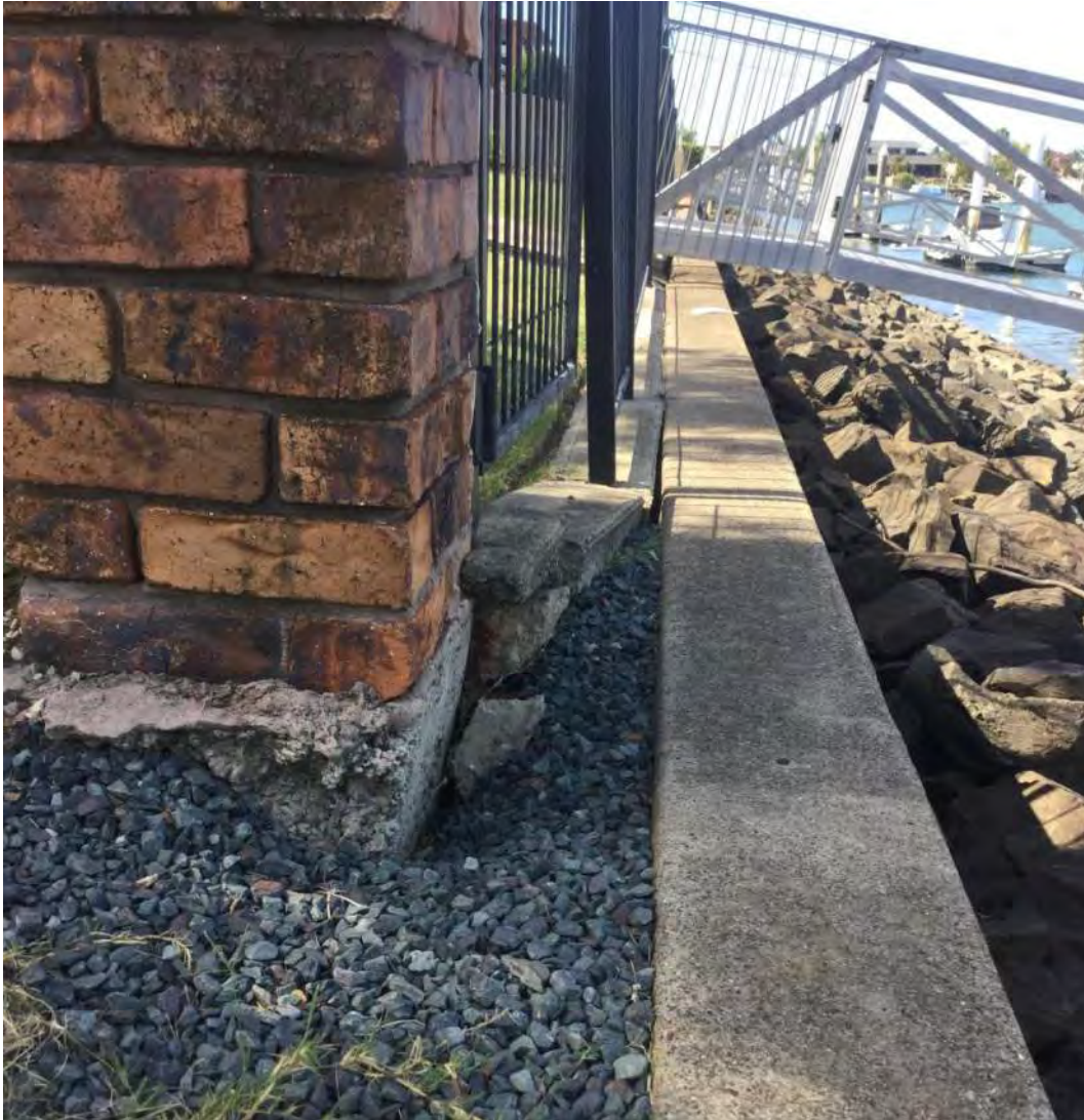
Figure 23: Sternlight Court boundary between 7-9 and 11 - Pre-construction view looking north, dated 25 January 2017
