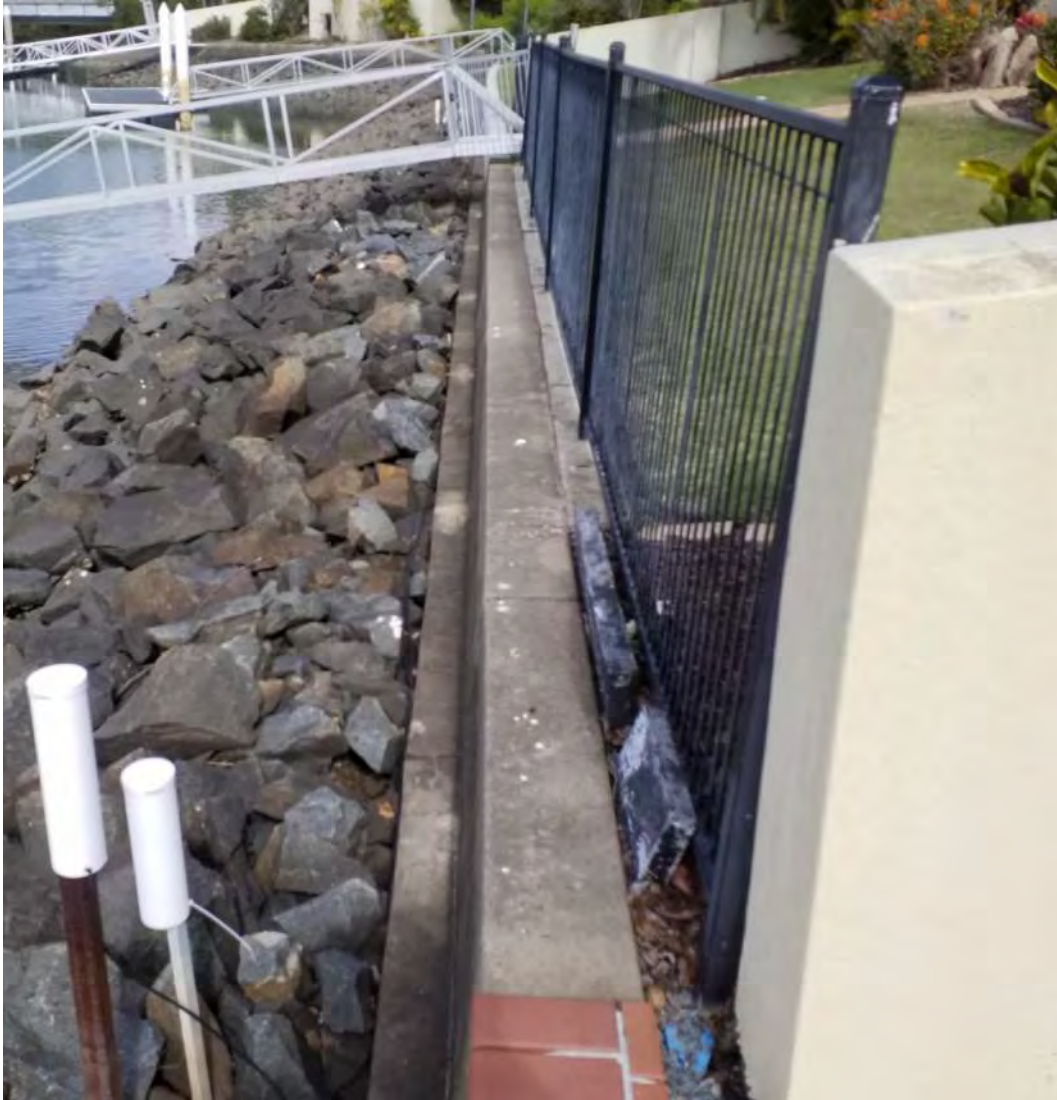
Figure 26: 11 Sternlight Court - Post-construction general view looking south, dated 20 June 2018 (from [12])
