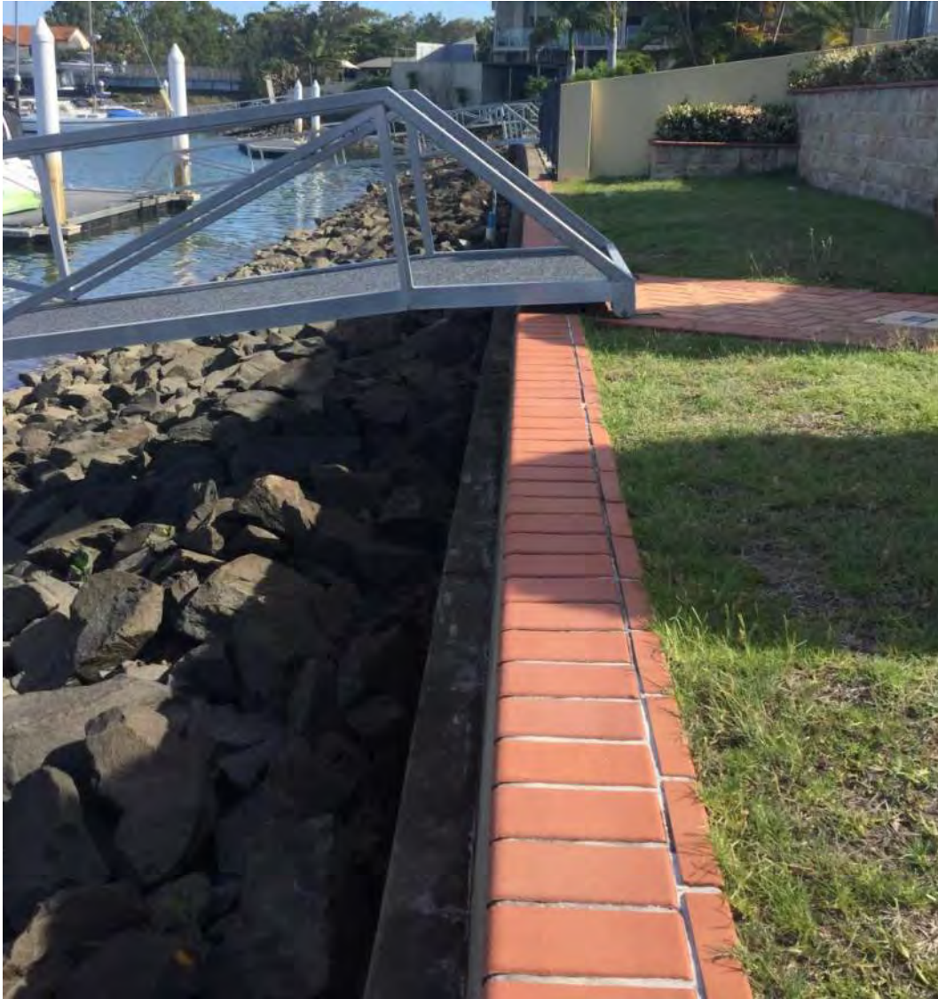
Figure 27: 13 Sternlight Court - Pre-construction general view looking south, dated 25 January 2017
