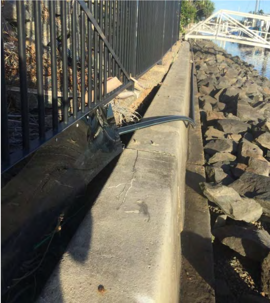
Figure 37: 83 Masthead Drive - Pre-construction general view looking east, dated 25 January 2017
