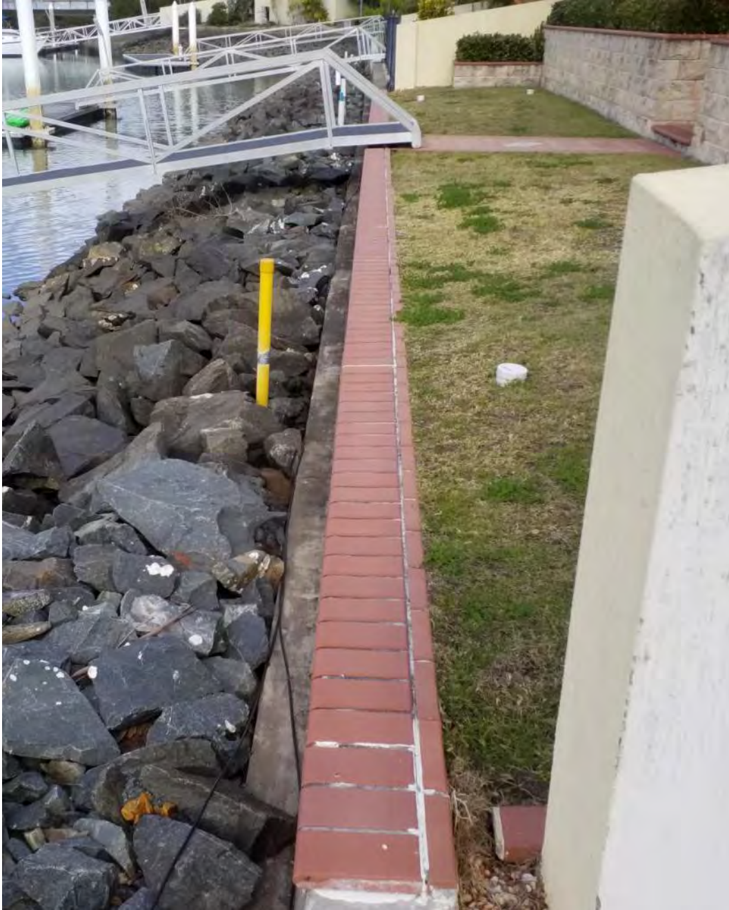
Figure 28: 13 Sternlight Court - Post-construction general view looking south, dated 20 June 2018 (from [12])
