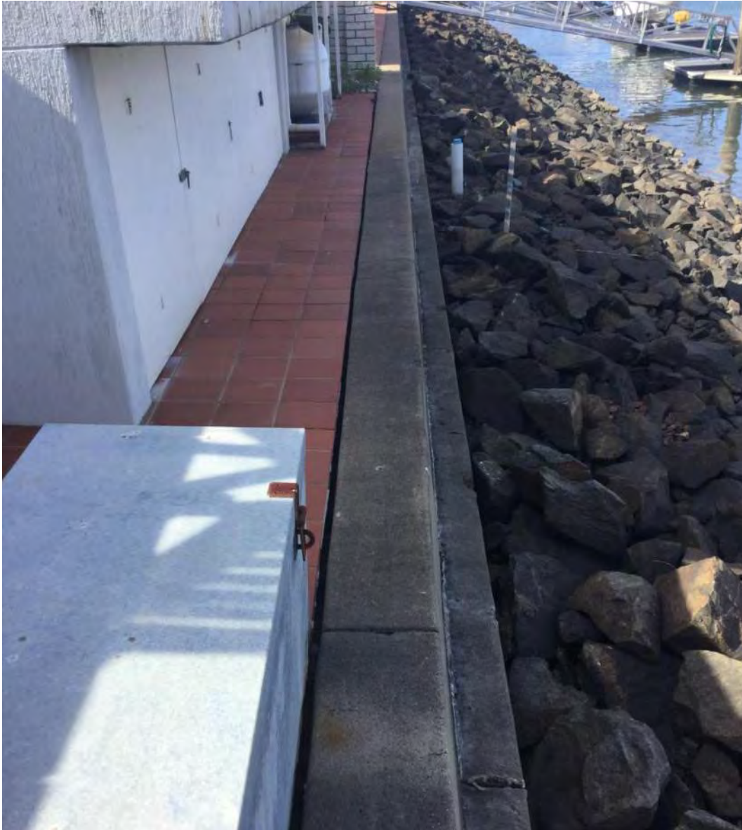
Figure 32: 15 Sternlight Court - Pre-construction general view from pontoon walkway looking north, dated 25 January 2017
