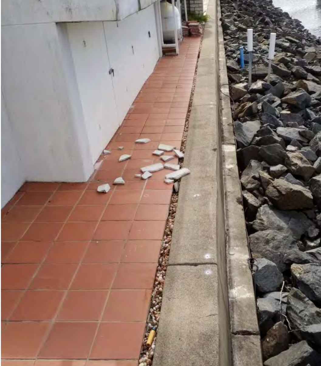
Figure 34: 15 Sternlight Court - Post-construction general view from pontoon walkway looking north, dated 20 June 2018 (from [12])
