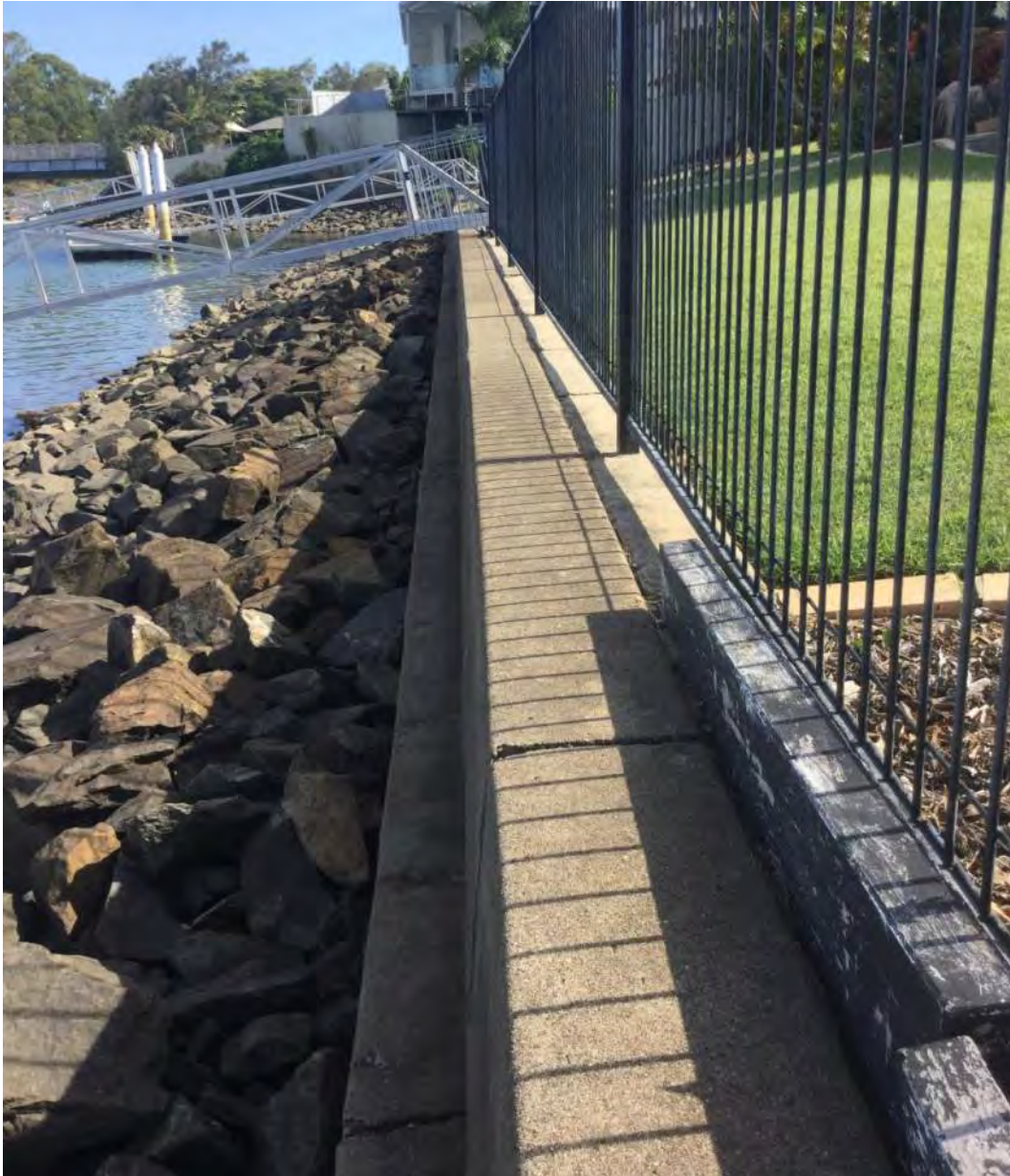
Figure 25: 11 Sternlight Court - Pre-construction general view looking south, dated 25 January 2017
