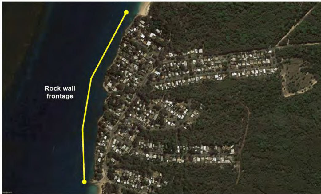
FIGURE 3-8 CENTRAL REACH – ROCK WALL FRONTAGE
