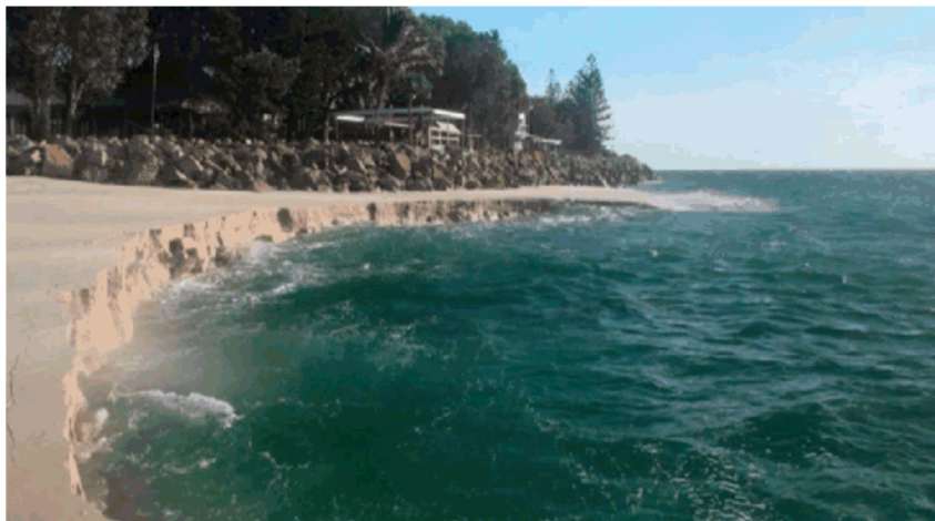
Figure 2-1 A Retrogressive Flow Slide Underway at Amity Point
