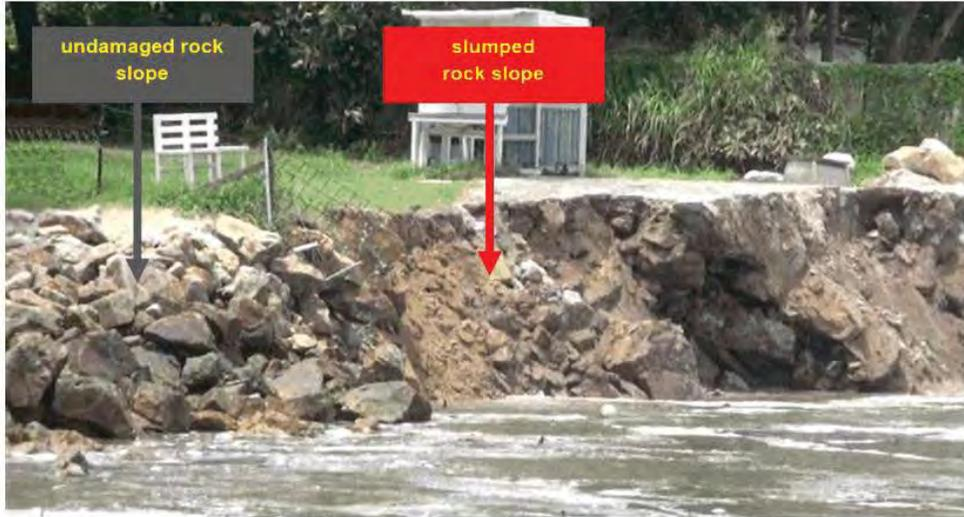
Figure 3-1 Emergency Tidal Works Trigger Event – Excessive Rock Slumping
