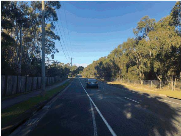
Plate 4 – View along McMillan Road looking east with Squirrel Glider Conservation Area on the right.
