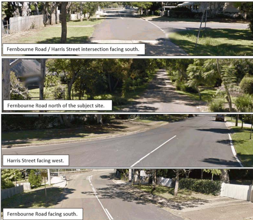
FIGURE 3.1 – IMAGES OF THE LOCAL ROAD NETWORK
