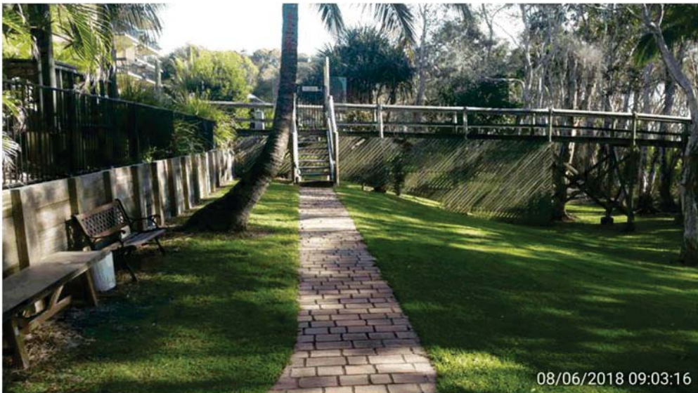
Figure 3 - footpath to board walk
