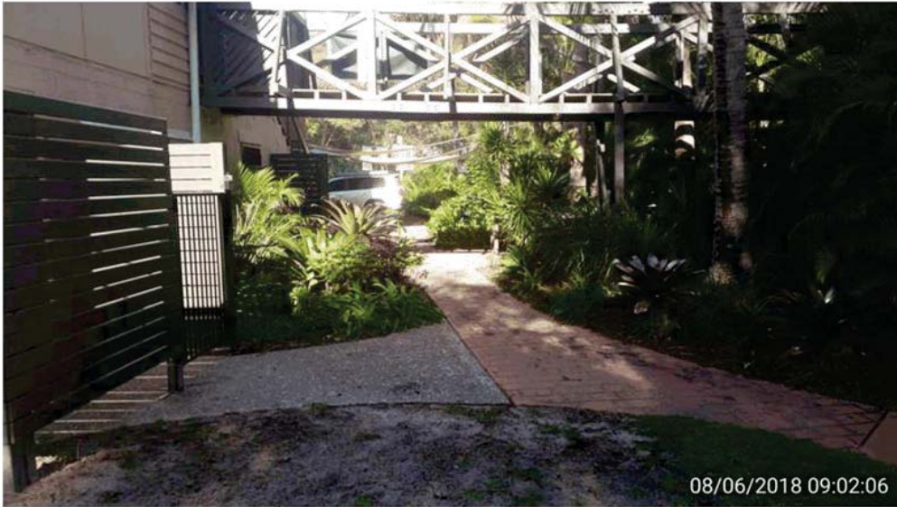
Figure 2 - public access from rear of the Anchorage Apartments
