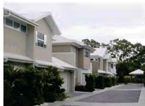
Parking integrated into the building design. Varied materials for access road punctuates and visually shortens the length of the access road. Change in materials can act as a traffic calming device
