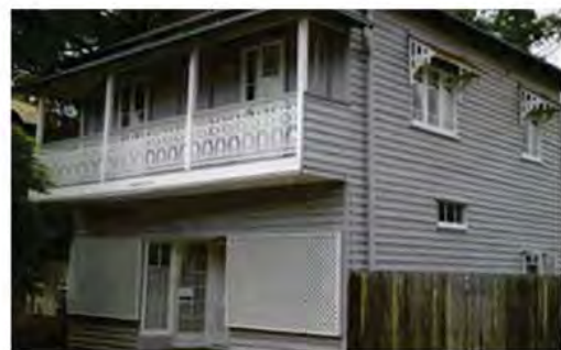
First floor projection Operable windows maximize natural ventilation and prevailing bay breezes Chamfer board wall cladding
