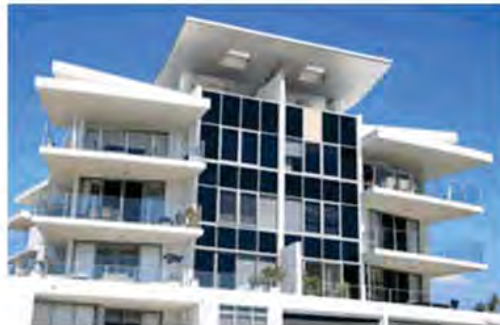
Dual aspects apartments, with doors and windows that can be opened, maximize natural ventilation opportunities. Common life areas have natural light.
