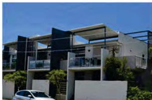
Elevated eaves creates shading and captures cooling breeze plus breeze filtered through screens at entrance and circulation points between the dwelling units.
