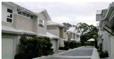
Figure 7 The site is arranged in a rectangular format, the house patterns display a variety of projections and articulation, and the garages are generally recessed so as not to dominate the street.
