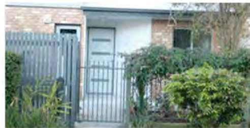
Figure 5 Each frontage unit has direct pedestrian access to the street. Combination of timber fencing and metal railing allows for privacy to courtyards plus transparency for access
