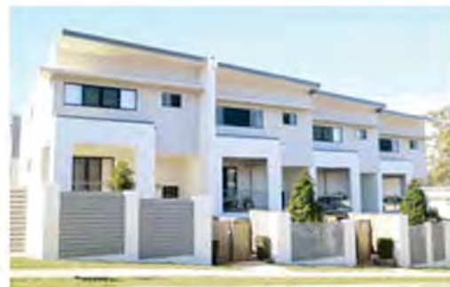
Building articulation, casual surveillance and direct entry to the street, all contribute to the streetscape
