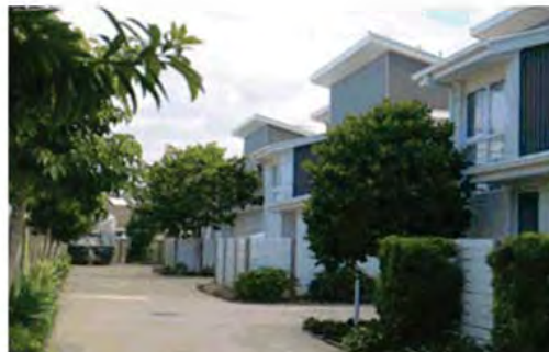
Staggered building alignment and landscaping reduces the visual impact of the internal road.
