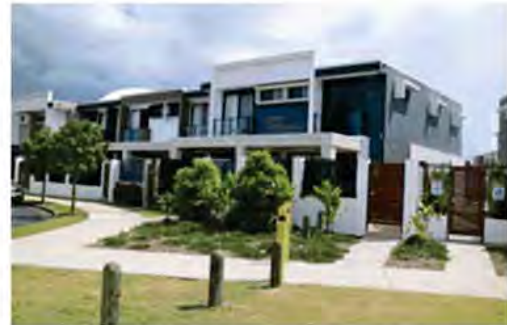
Front doors addressing the street.
