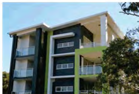
Pitched roof form and articulation breaks down the scale of an apartment building
