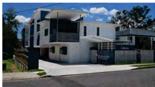
Refuse storage located within the site and with screening and good ventilation.
