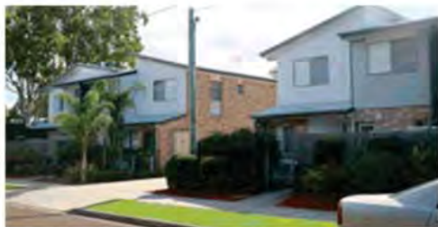
Figure 4 Varied depth of facade and articulation of roof line together with the cohesive palette of brick, render and light weight cladding creates an interesting streetscape.
