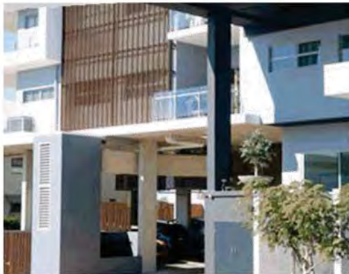
Plant and services screened but still allow for easy access for maintenance and inspection. Services screened to blend in with overall design and simple palette of colours of building.
