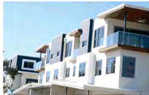
Balconies can still add outdoor living space and visual feathering at key corners, with a textured and articulated facade to a west facing elevation
