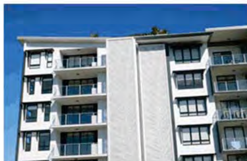
This apartment block has a north eastern aspect. The artistic screening provides a distinct identity and gives vertical emphasis to break up the long facade.
