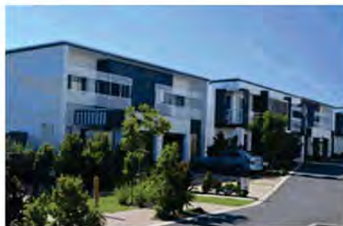
Shared access with garages set back beneath housing helps to reduce the footprint of car parking at ground level and visual impact.
