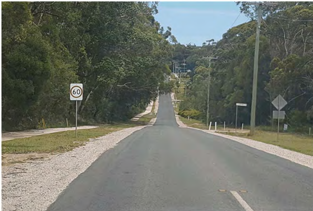
Photograph 9: Westbound view along Minjerriba Road from the Centre Road intersection (Segment 1).
