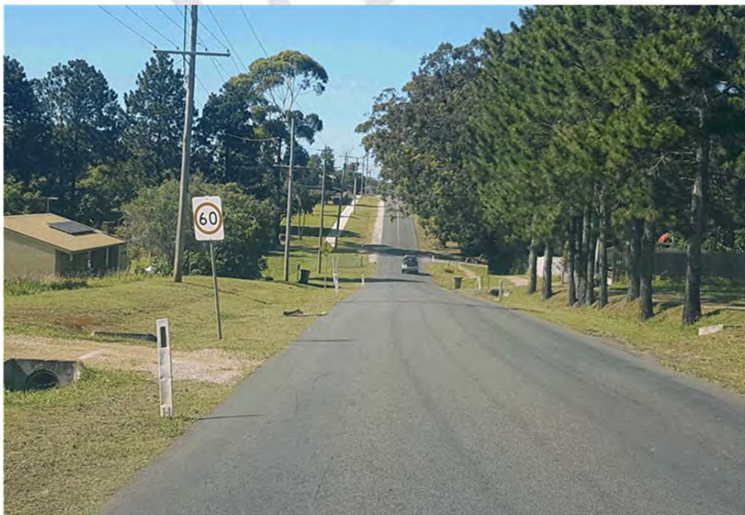
Photograph 6: Southbound view on High Street at the Bernborough Street intersection (Segment 2).
