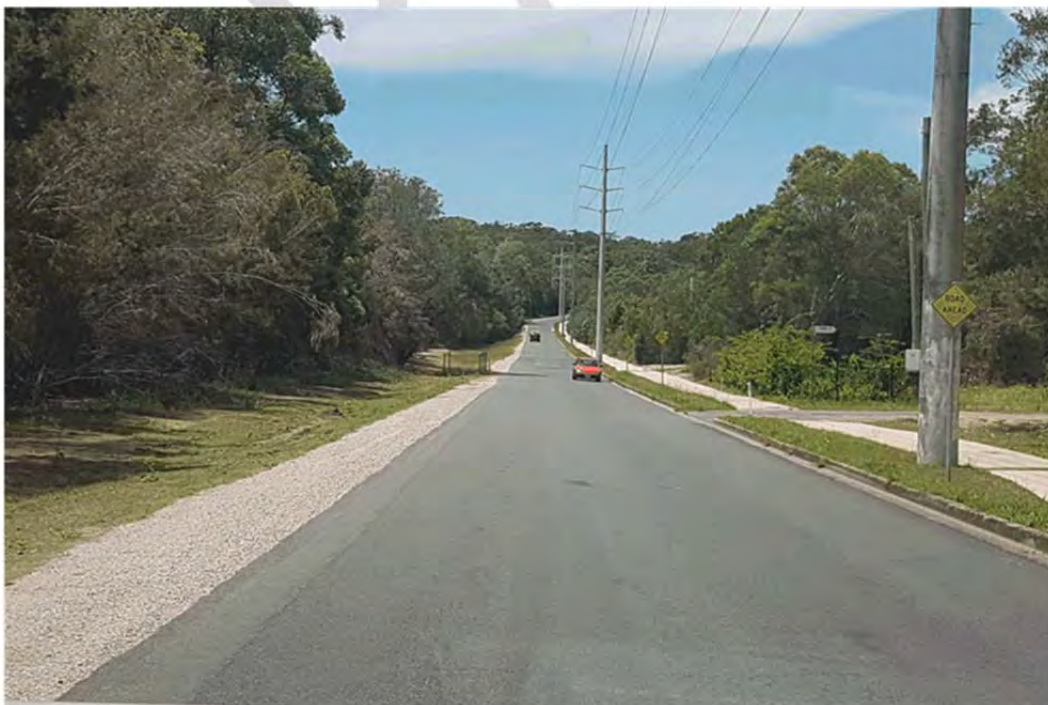
Photograph 2: Southbound view along Centre Road south of the Davidson Road intersection.
