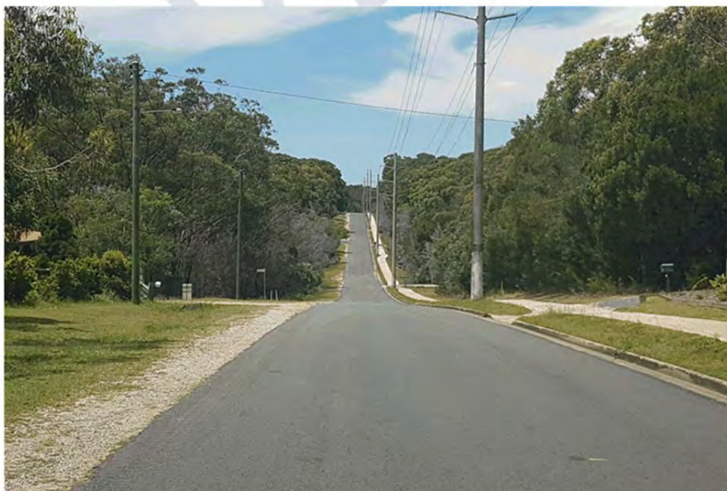
Photograph 4: Southbound view along Centre Road north of the Gay Terrace intersection.
