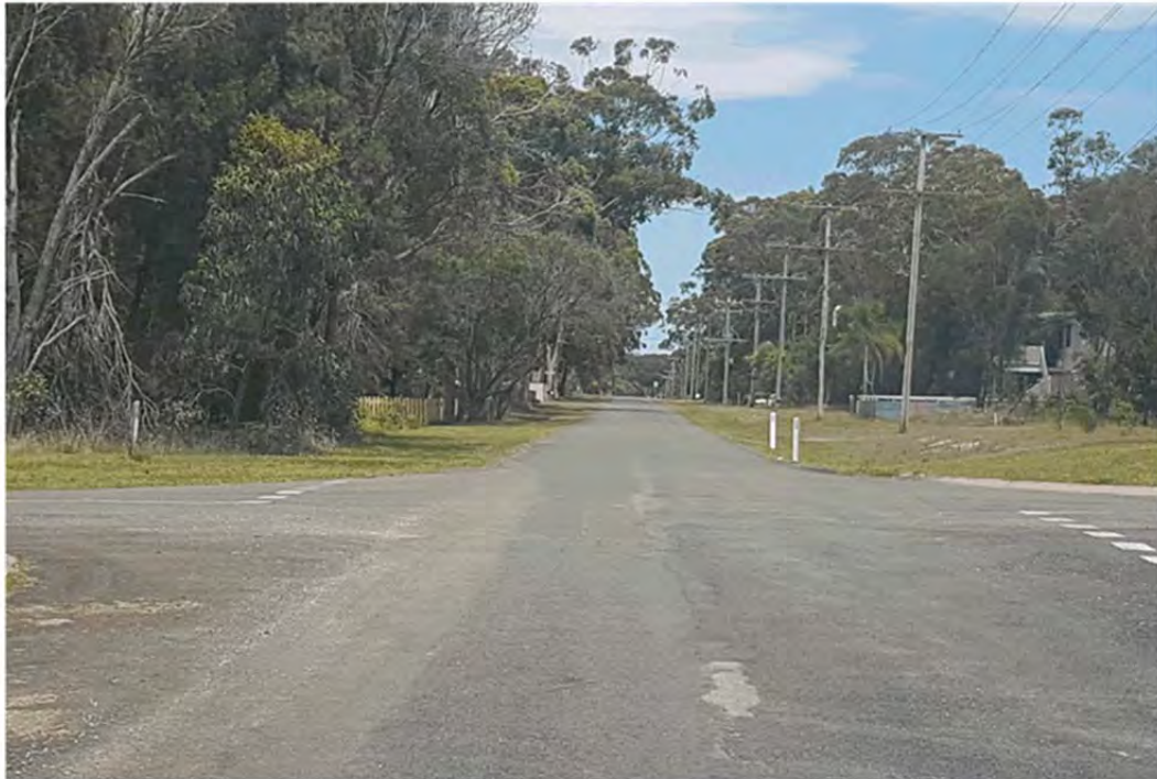
Photograph 7: Westbound view along Minjerriba Road from the Jasper Street intersection (Segment 2).
