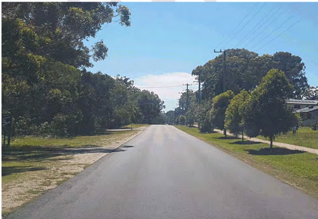
Photograph 2: Eastbound view on Canaipa Road west of the Hawthornden Drive intersection (Segment 1).
