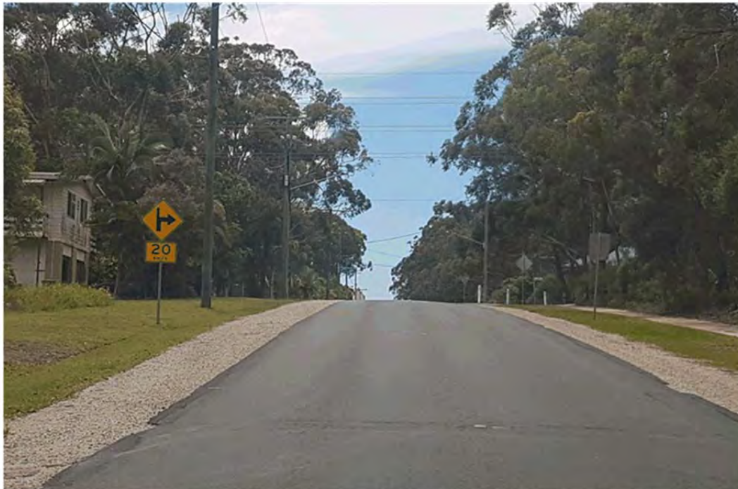
Photograph 3: Eastbound view along Minjerriba Road on approach to Centre Road intersection (Segment 1).
