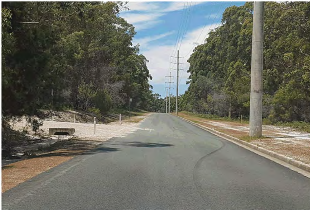
Photograph 7: Southbound view along Centre Road south of the Cunningham Avenue intersection.
