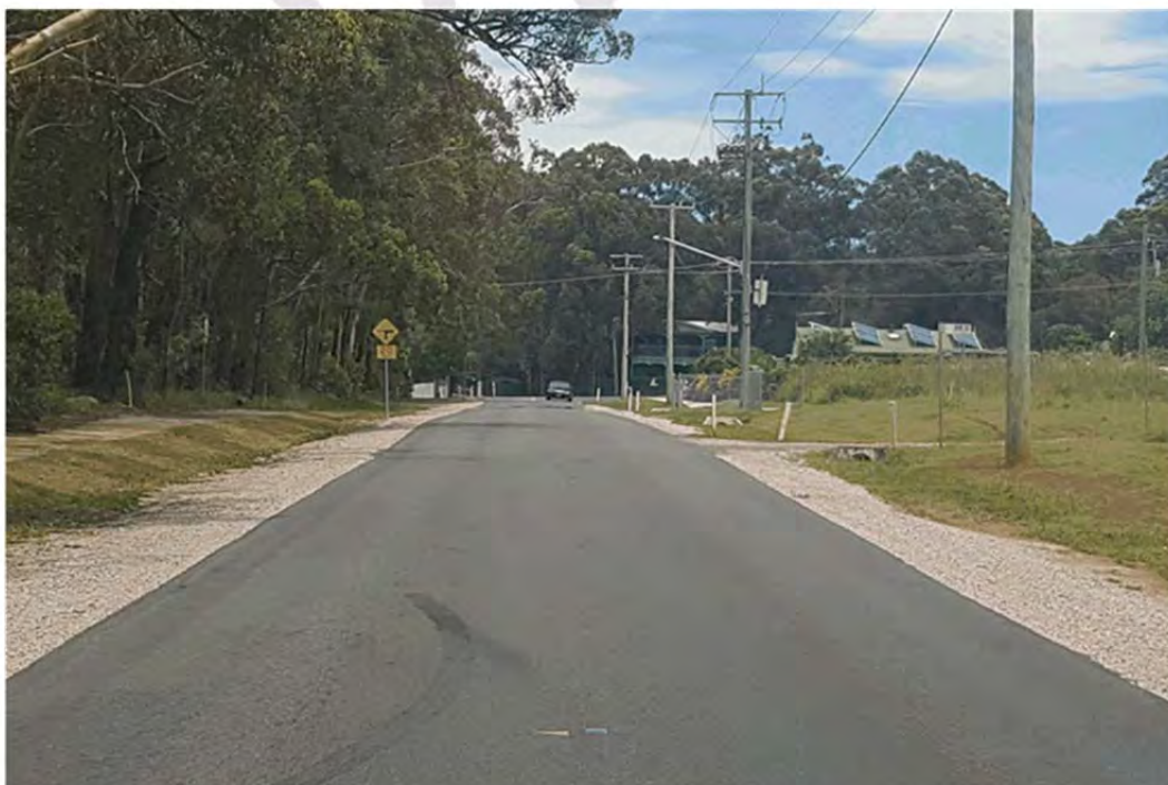
Photograph 10: Westbound view along Minjerriba Road near the Oak Street intersection (Segment 1).
