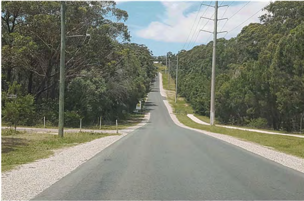
Photograph 1: Southbound view along Centre Road south of the Minjerriba Road intersection.
