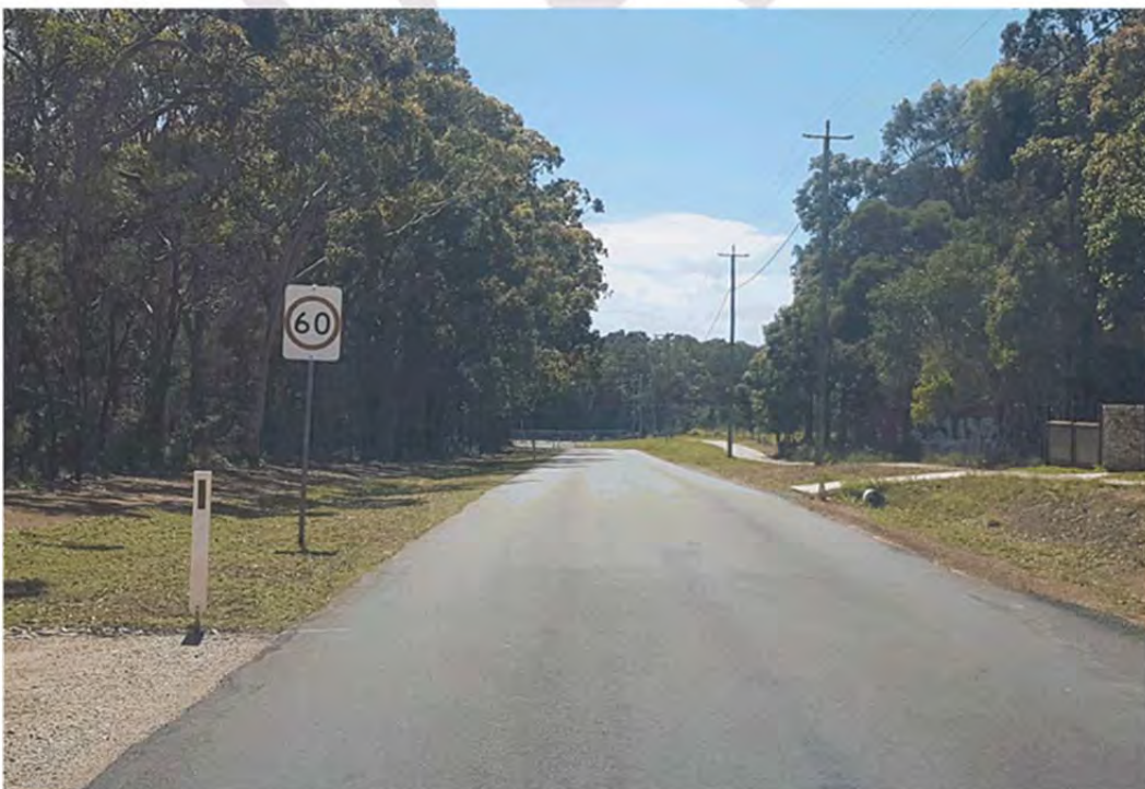
Photograph 4: Eastbound view on Canaipa Road east of the Cestrum Street intersection (Segment 1).
