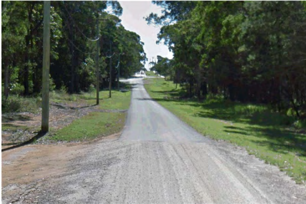
Photograph 9: Northbound view on High Street at the Titania Terrace intersection (Segment 3).
