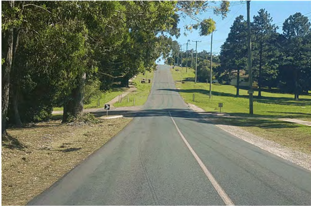
Photograph 11: Northbound view on High Street north of the Pharlap Street intersection (Segment 2).
