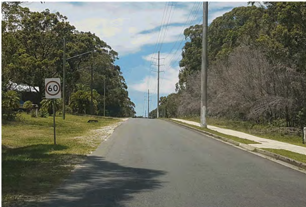
Photograph 5: Southbound view along Centre Road south of the Hume Street intersection.
