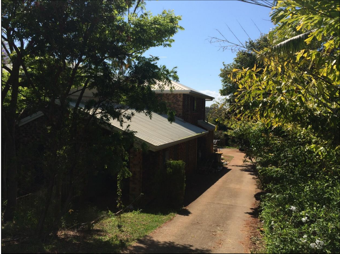
Photo 1: View of existing dwelling at 7 Fernbourne Road, Wellington Point.
