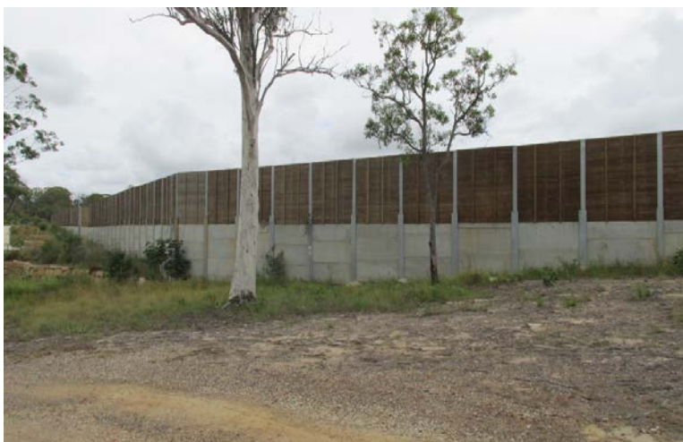
Figure 4 – View of the edge area looking north from the core area.
