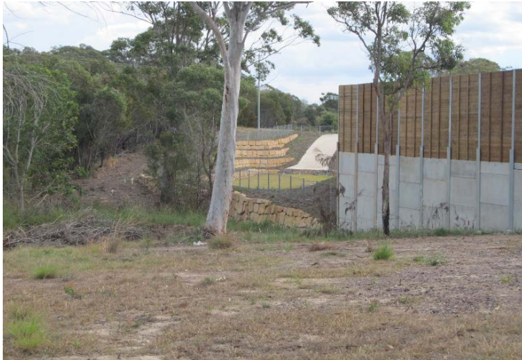
Figure 5 – View of the edge area looking west from the core area.
