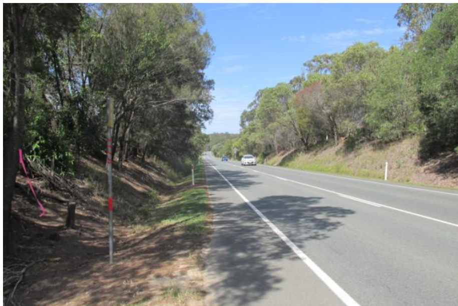
Plate 5. Redland Bay Road.
