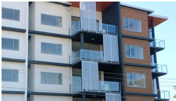
Figure 11 Design includes lattice operable screens, prominent vertical columns, composite timber cladding to the walls and exposed eaves. All units have private open space that achieves natural light. Each unit has dual aspect to promote cross ventilation.
