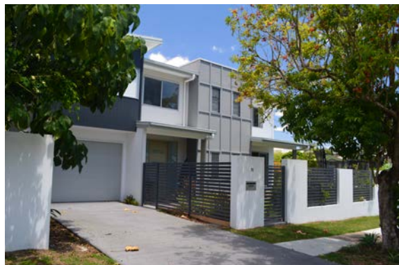
Fencing materials allow for casual surveillance whilst also maintaining privacy for residents.
