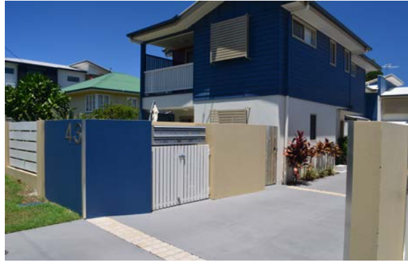
Service boxes integrated into the colour palette of the scheme.
