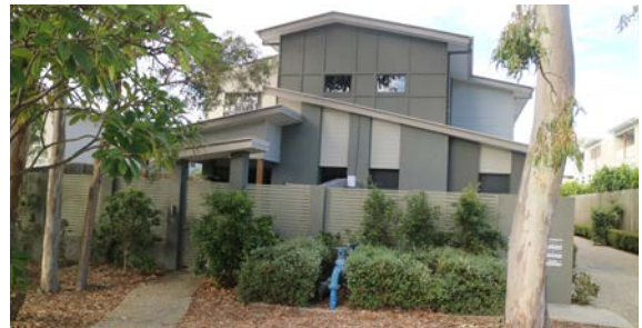
Figure 2 Building facade articulation, varied skillion roof form and mixed material fencing provide interest to the street. The complementary material and colour palette of the built structures are softened by vegetated landscaping. The street interface could be improved by lower or semi-transparent fencing.
