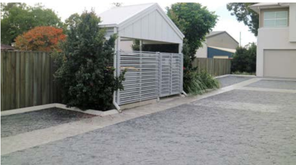
Multiple services screened within the design.
