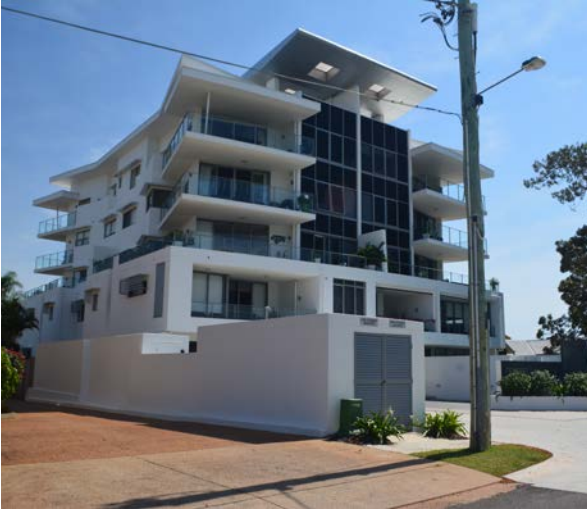
Services and plant need to be easily accessible for maintenance but can be designed to blend in with overall design and simple palette.
