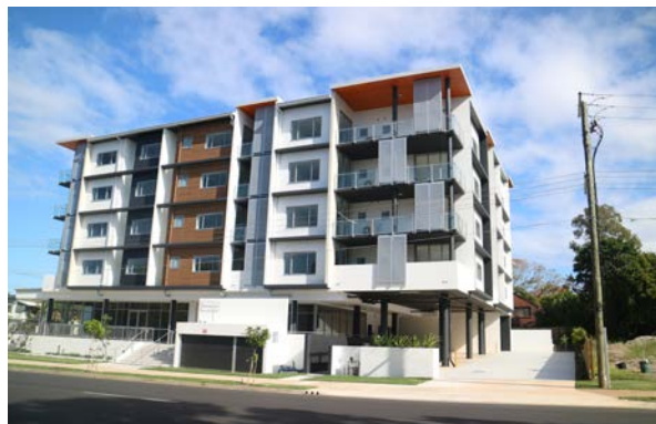
Dwellings with east facing aspects can also benefit from angled roofs, overhanging eaves and screens.
