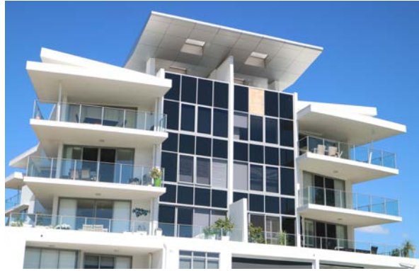
Dual aspect apartments, with doors and windows that can be opened maximise natural ventilation opportunities. Common lift areas have natural light
