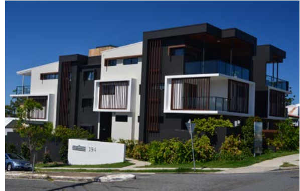
A well proportioned building with strong articulation addresses the corner.
