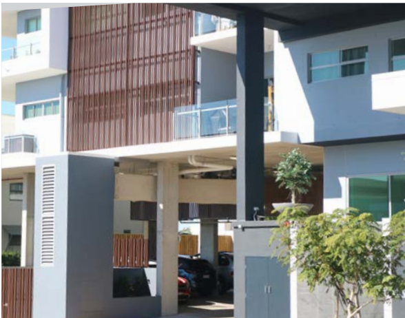
Plant and services screened but still allow for easy access for maintenance and inspection. Services screened to blend in with overall design and simple palette of colours of building.
