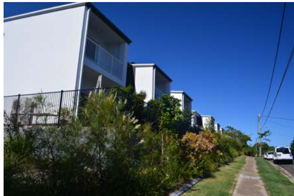
Railings with landscaping provide transparency to the street, the raised aspect provides an amount of privacy.
