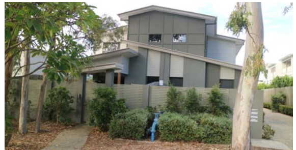
Figure 2 Building facade articulation, varied skillion roof form and mixed material fencing provide interest to the street. The complementary material and colour palette of the built structures are softened by vegetated landscaping. The street interface could be improved by lower or semi-transparent fencing.
