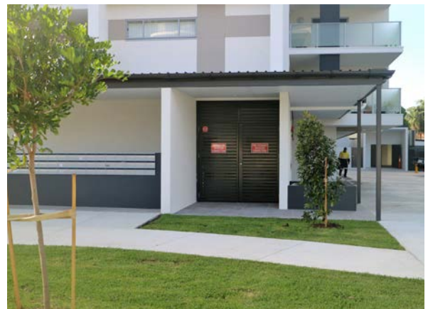
Services and plant discreetly housed near mail boxes.
