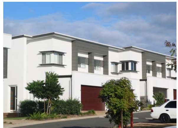
Variation in building depth, hoods, projections and screening provides solar access and effective shading
