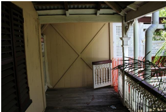
Figure 26: View to residential extension from north verandah of original house, note the cross bracing.
