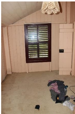
Figure 22: Enclosed former verandah, room next to lounge room.
