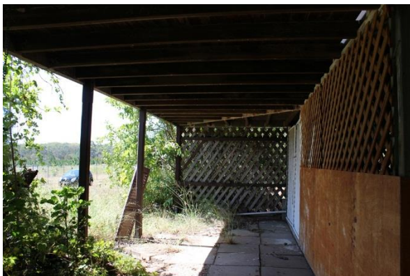
Figure 33: Underneath verandah at western side of residential extension.
