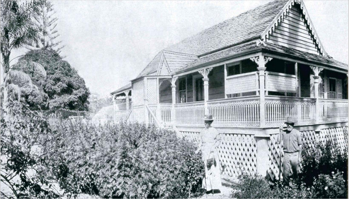
Figure 5: Side and front view of the house, showing ornamental gardens, c.1890s. Note that the building has been extended and demonstrates the addition of a range of period embellishments including iron balustrading, fretwork, and lattice (Howells 2000).
