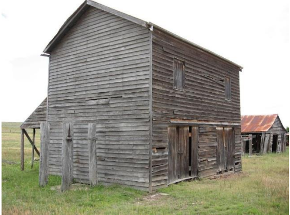
Figure 94: Castleholme outbuildings in 1979 (EHP).
