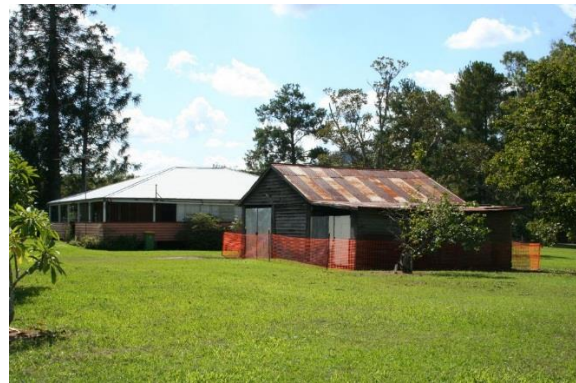
Figure 91: Bankfoot house from the southwest (EHP 2007).
