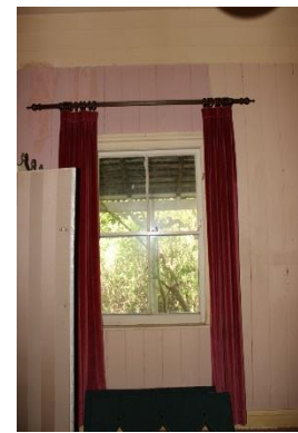
Figure 25: Window in main bedroom.
