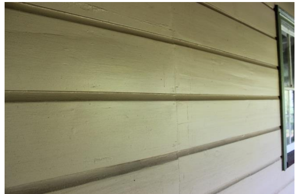
Figure 18: Detail of timber chamferboard cladding at verandah (front) of original house.
