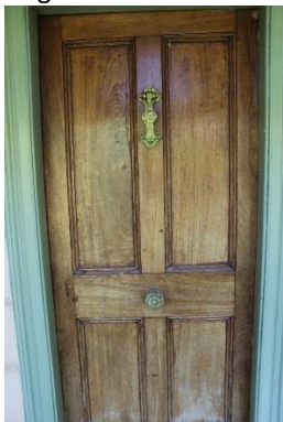
Figure 16: Front entrance door to original house.
