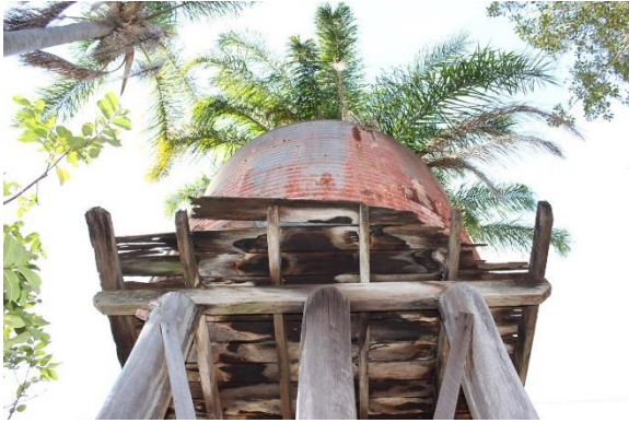
Figure 65: Looking up at the tank, standing at the base.
