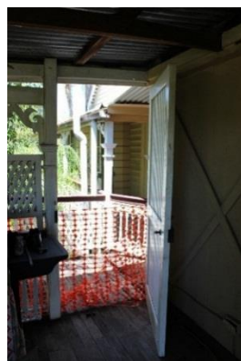
Figure 29: Verandah door to northern stairs at residential extension.
