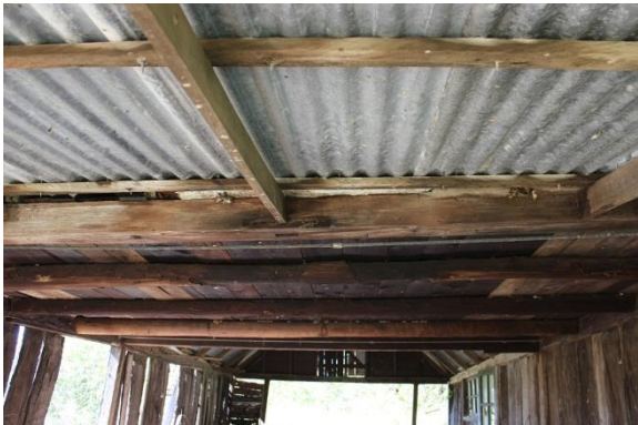
Figure 62: Flat section of ceiling at garage.
