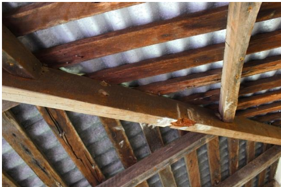
Figure 14: Shingle battens on east verandah at original house.
