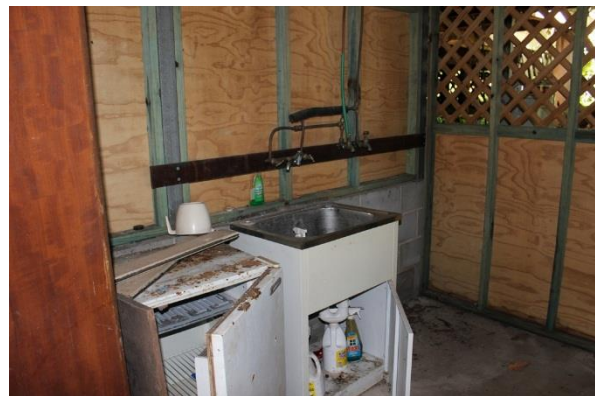
Figure 34: Modern laundry under residential extension.
