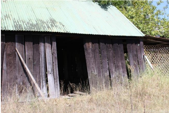
Figure 57: Slab timber walls of the garage.
