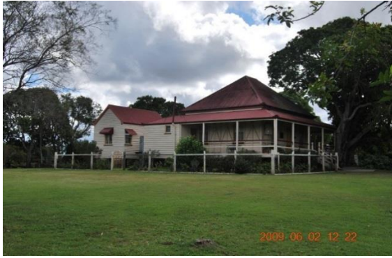
Figure 88: Mayes Cottage (EHP 2016).
