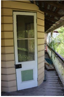
Figure 19: One of two doors at bay window.
