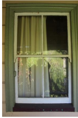
Figure 20: Double hung window at lounge room, seen from front verandah.
