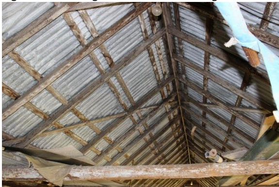
Figure 45: Ceiling of milking shed.
