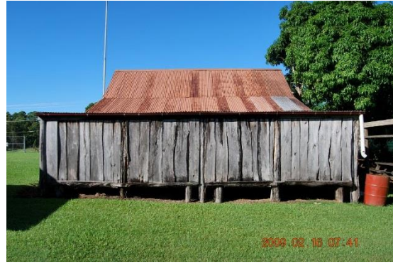
Figure 96: Slab barn – recently rebuilt (EHP).
