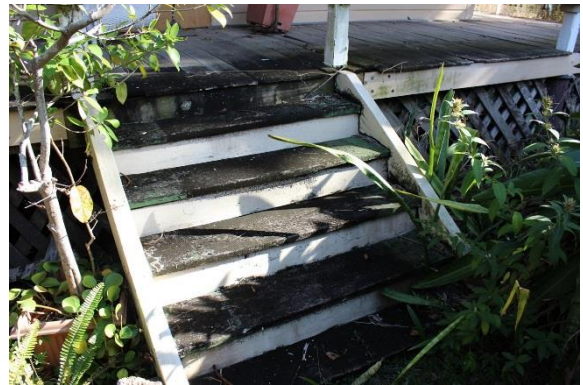
Figure 15: Front stairs and adjacent lattice.
