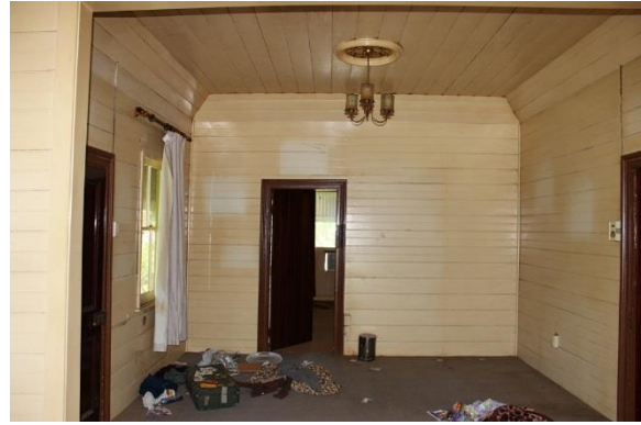
Figure 21: Lounge room and door leading to main bedroom (centre of image). Note coved, boarded ceilings.
