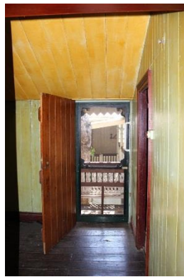
Figure 23: Enclosed former verandah and back door leading to verandah and extensions.
