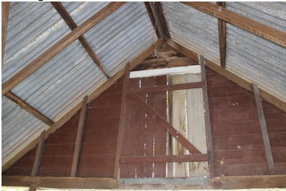
Figure 61: Pitched section of the ceiling of garage, and door in gable.
