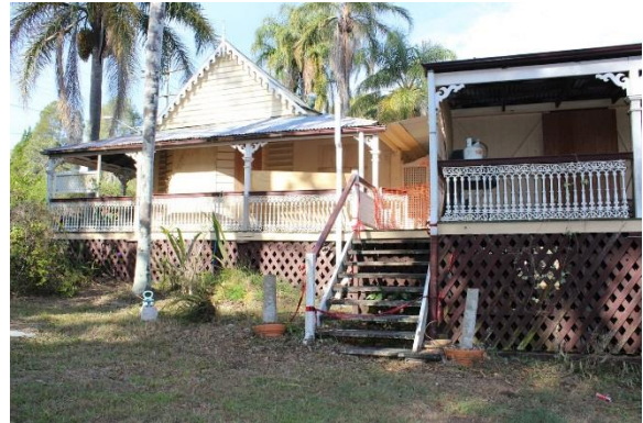
Figure 83: Side of house cleared of non-significant and invasive vegetation, including two Brazilian cherry trees (either side of stairs) that were growing in plastic pots but had rooted into the ground.
