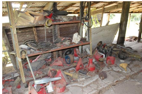
Figure 48: Equipment stored in milking shed at time Council purchased the farm complex.
