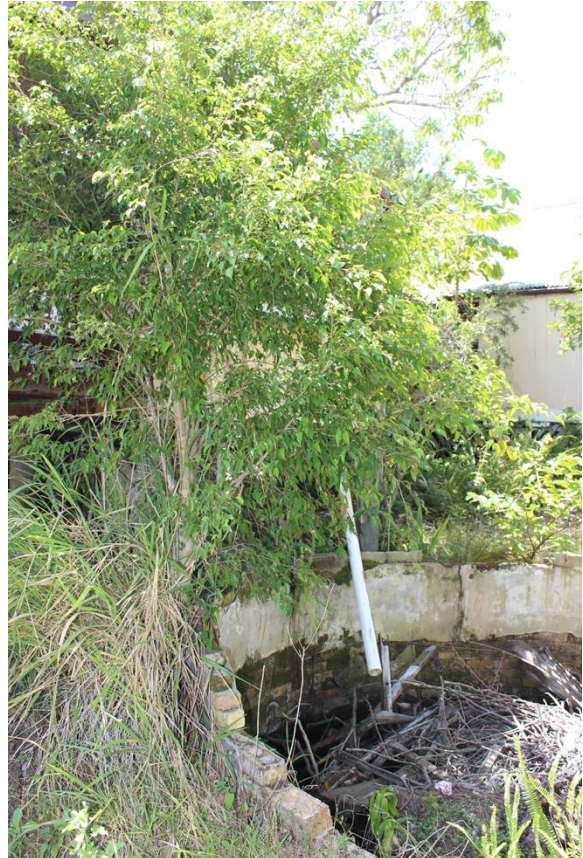
Figure 68: Brick tank adjacent to kitchen.
