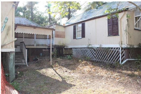
Figure 84: After clearing of mango and callistemon trees next to the house, removed due to proximity to structure and observed impacts on foundations.
