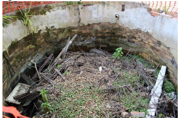
Figure 70: Inside brick cistern, after external vegetation clearing.
