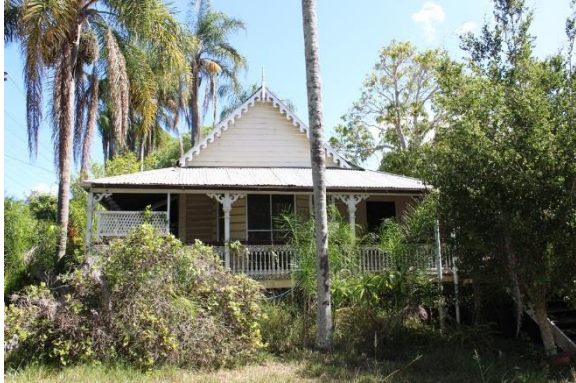
Figure 12: Side (north) view of the original house prior to excess vegetation removal.
