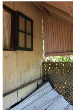
Figure 55: Under annex at cream shed.
