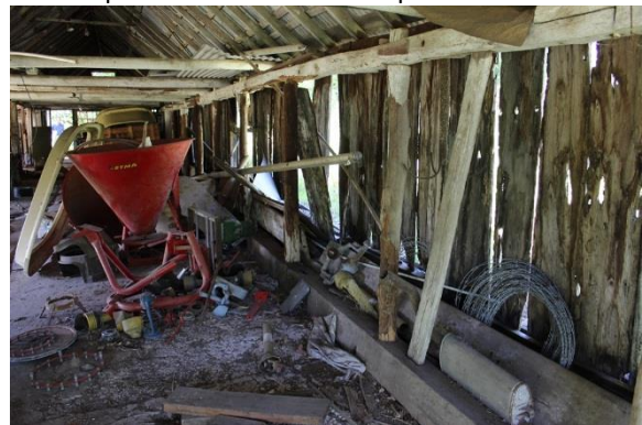
Figure 50: Slab wall and cow bales.
