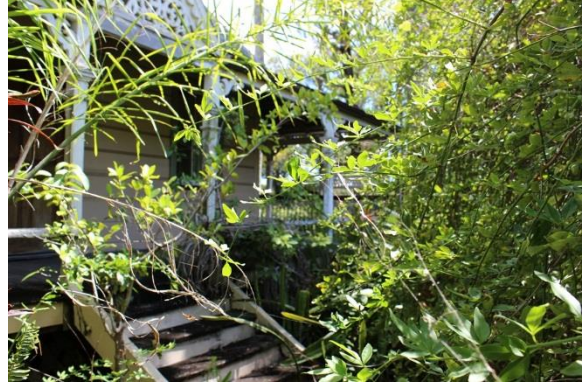
Figure 75: Overgrown vegetation at front of house, obstructing the front entrance.
