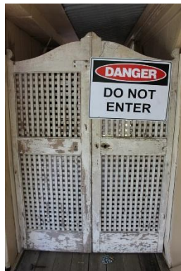
Figure 17: Privacy gate at passage between original house and residential extension.
