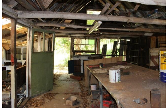
Figure 44: Interior of milking shed, looking north.
