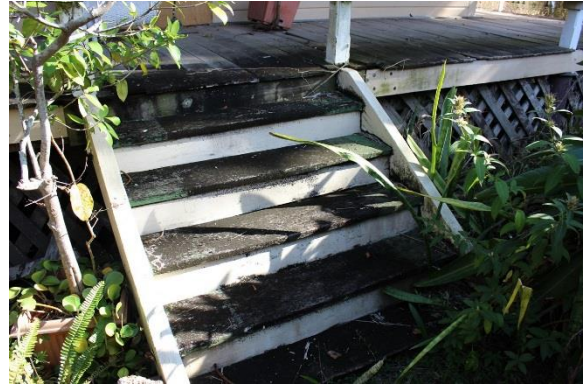
Figure 81: Front steps and surrounds now cleared of excessive vegetation.
