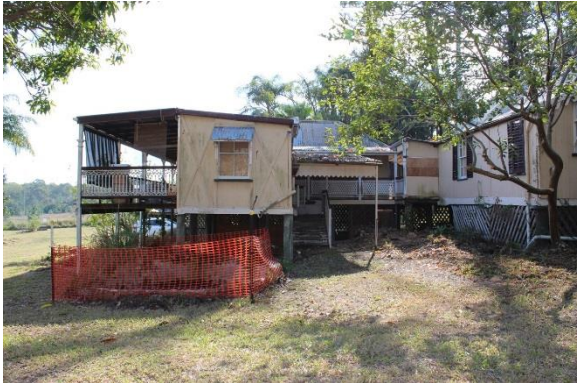
Figure 37: View of kitchen wing from the south – note cross-bracing and addition of verandah and roof over stairs.
