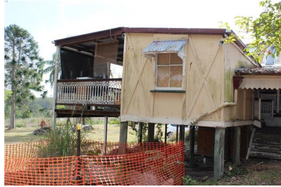
Figure 87: Clearing around brick cistern and securing off the area temporarily.
