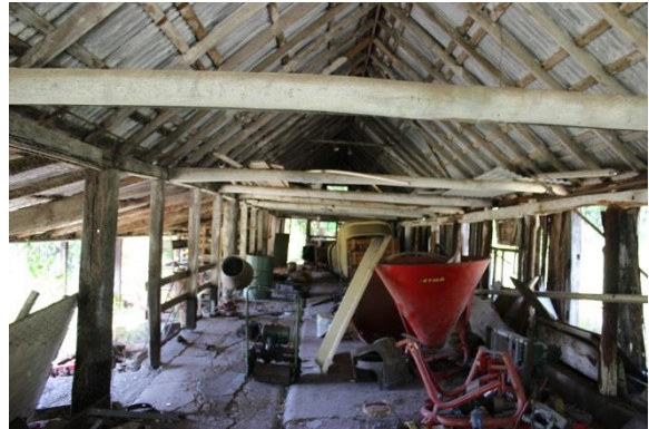
Figure 46: Interior of milking shed, near the cow bales – note skillion addition to west
