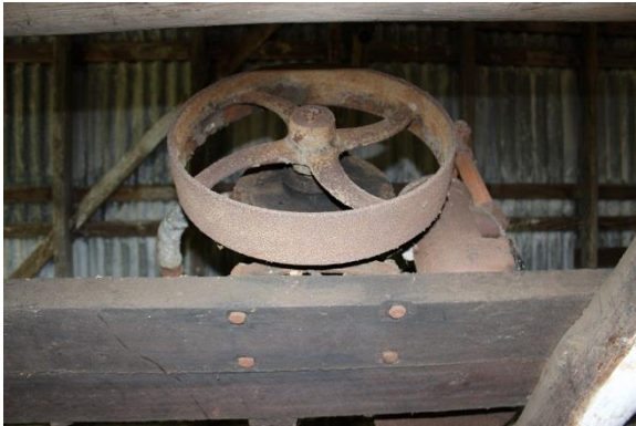
Figure 47: Original machinery in ceiling of milking shed.
