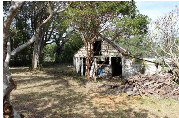
Figure 85: After slashing and trimming near the milking shed.
