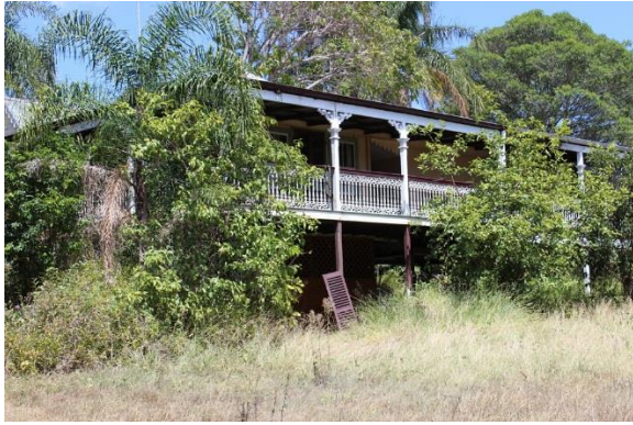
Figure 31: View to c.1980s verandah behind residential extension and kitchen from west.
