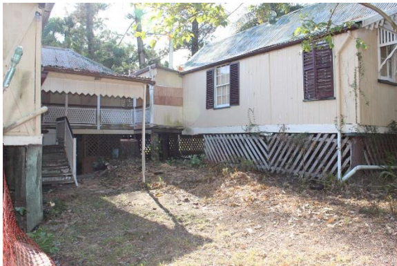
Figure 84: After clearing of mango and callistemon trees next to the house, removed due to proximity to structure and observed impacts on foundations.
