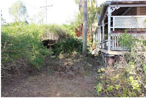
Figure 80: Front entrance now accessible. Still more clearing required. Note build-up of solid and humus at front of house.
