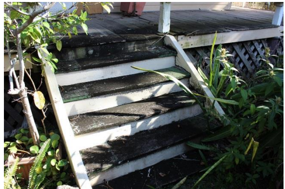
Figure 15: Front stairs and adjacent lattice.
