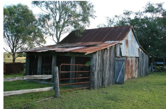
Figure 98: Horse shed in 2006 (EHP).
