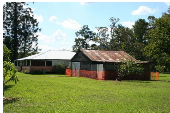
Figure 91: Bankfoot house from the southwest (EHP 2007).
