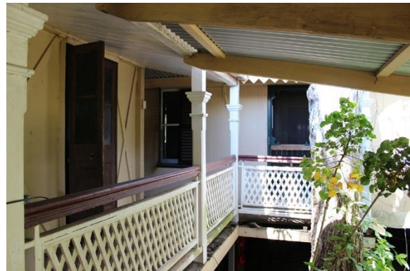
Figure 36: residential extension and verandah/covered walkway looking east from kitchen doorway. Note recent awning addition over kitchen stairs.
