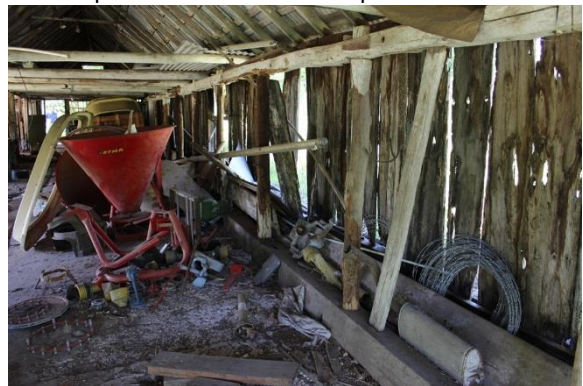
Figure 50: Slab wall and cow bales.
