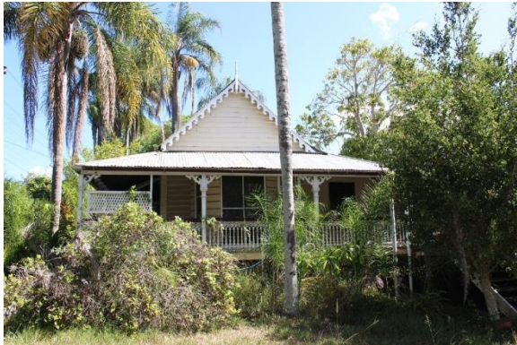
Figure 12: Side (north) view of the original house prior to excess vegetation removal.
