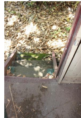
Figure 56: Steps leading into cream shed.
