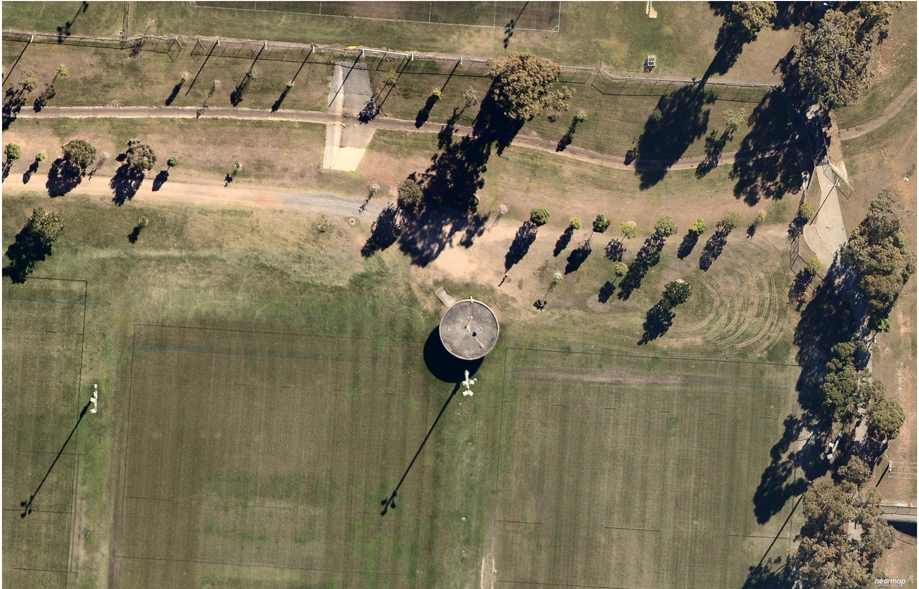
PS 6 Upgrade, 44 Smith Street Cleveland, Pre-construction, 7/7/14
