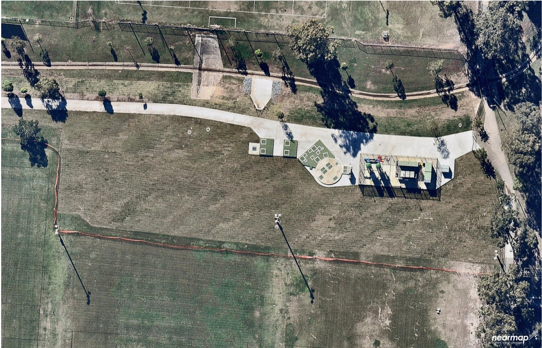
PS 6 Upgrade, 44 Smith Street Cleveland, Post-construction, 1/7/16
