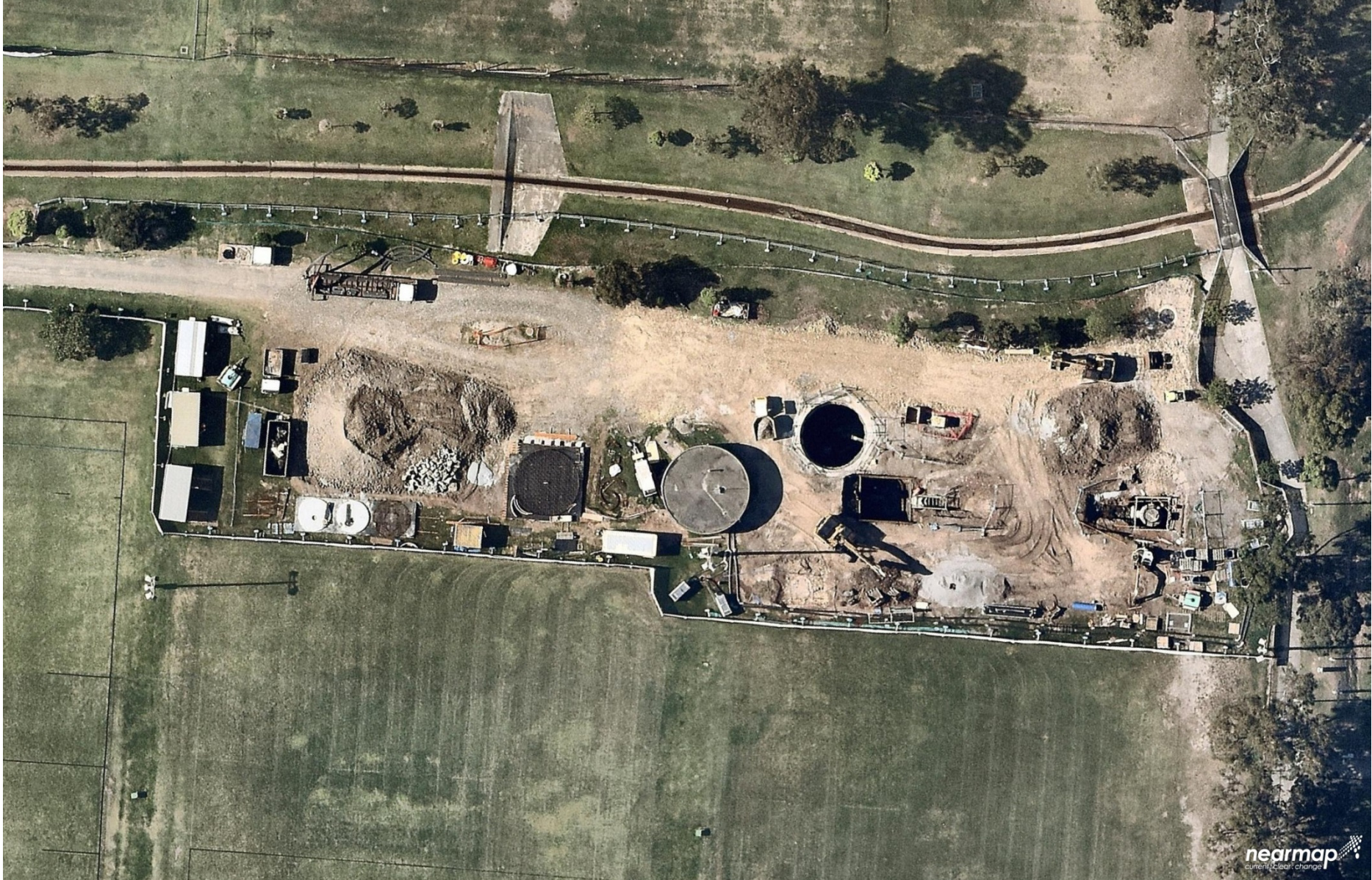
PS 6 Upgrade, 44 Smith Street Cleveland, Construction, 19/11/15
