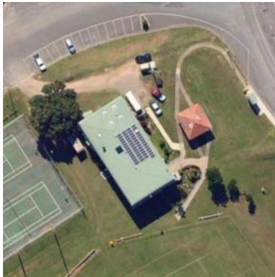
Image 2 – Aerial of clubhouse prior to building extension
