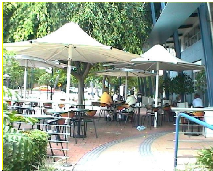
Photograph 6 – Tactile paving free of obstructions
