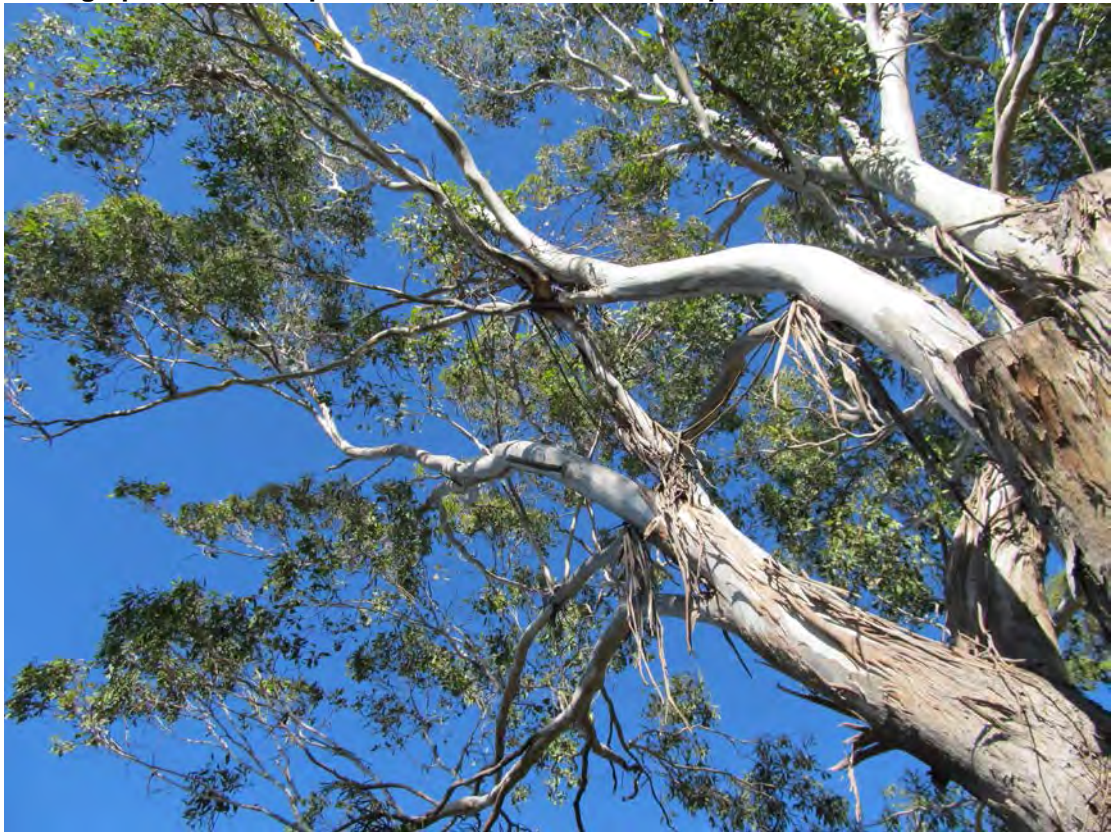
Photograph 5 – From all angles, tree 1 is of poor structural integrity and form.
