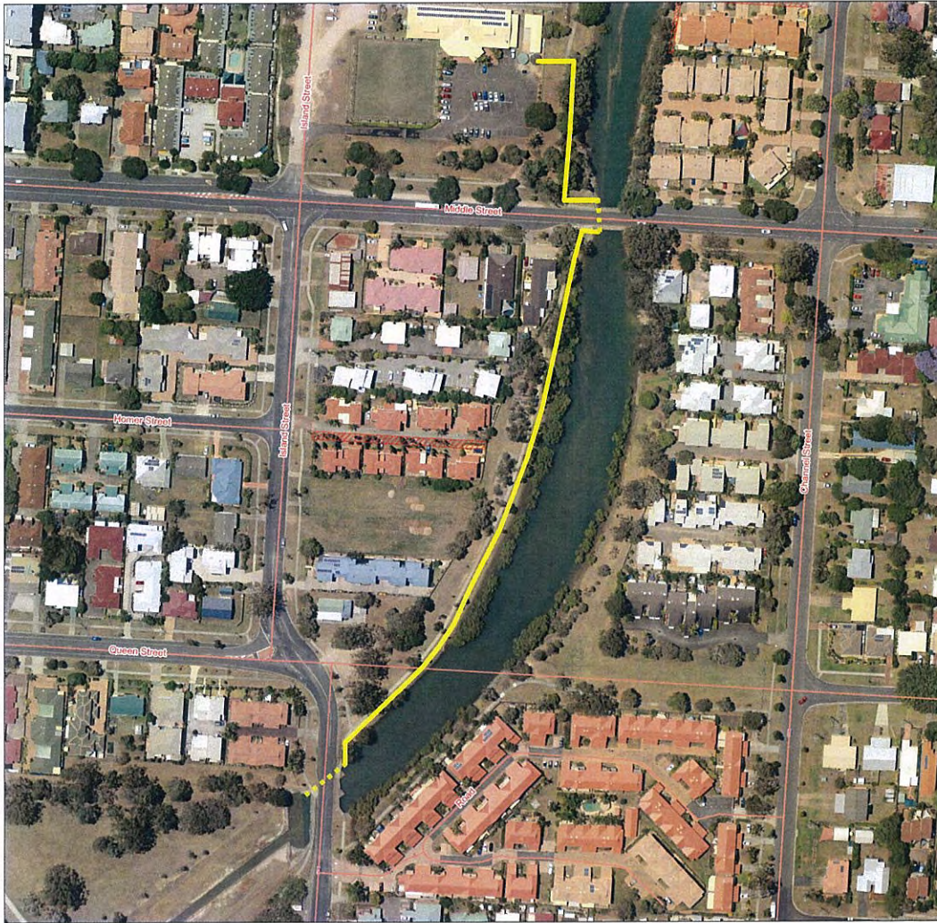
Island Street Pipe Crossing (Underneath Road)
