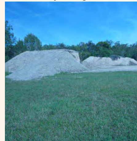
Road scalplings stockpiled at Redland Bay waiting to be reused
