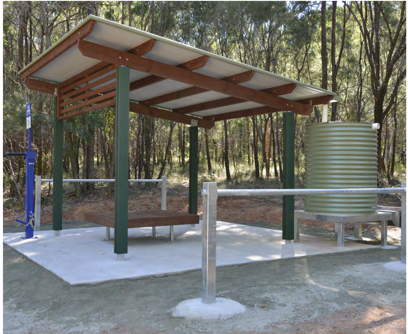
Figure 5: Days Road Trailhead Shelter
