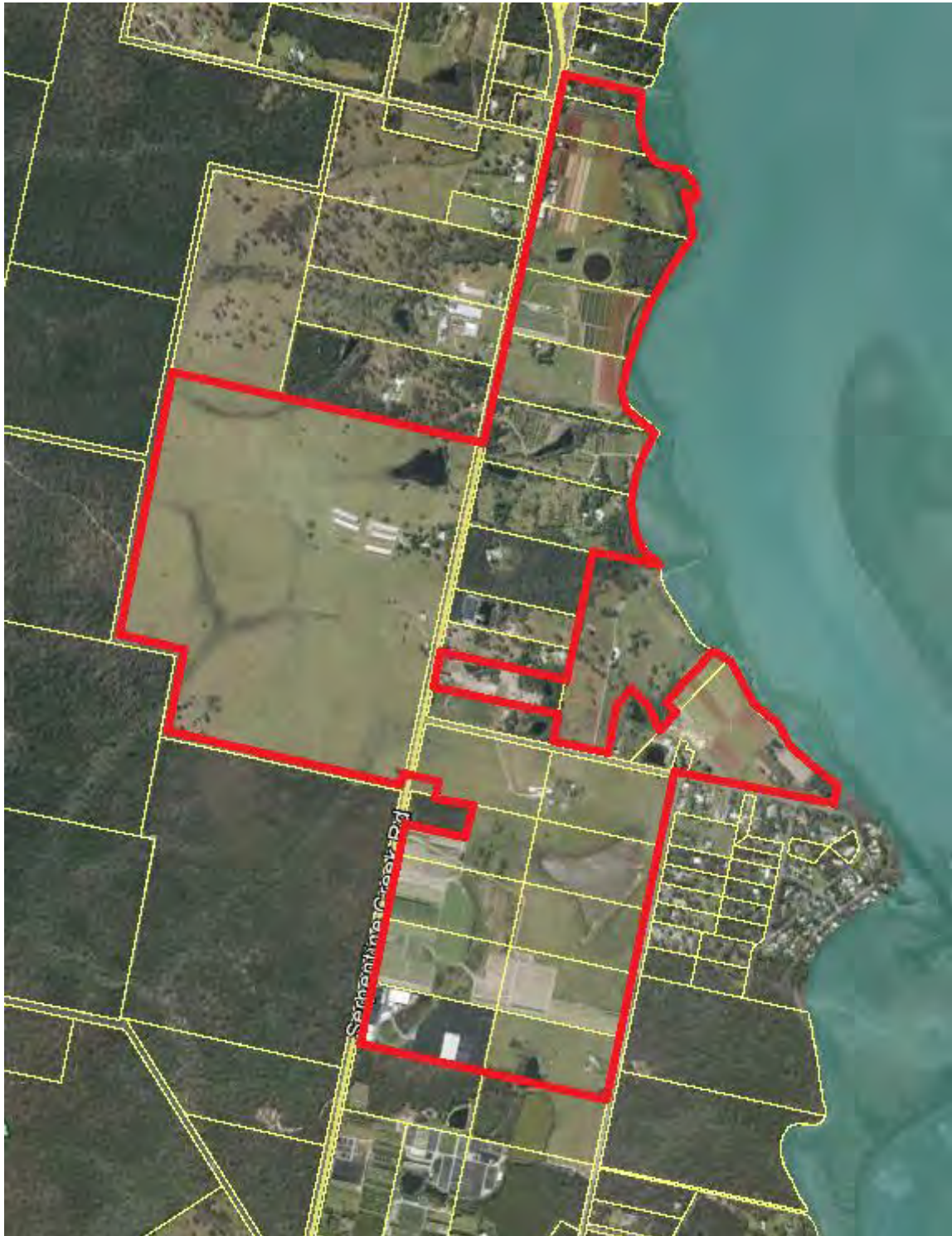
Figure 2 – Aerial Photograph of the Shoreline site showing extent of land to which the Shoreline POD applies
