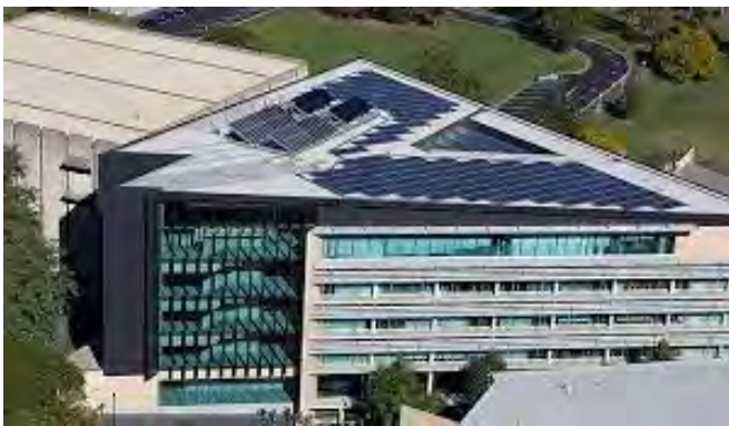
University of Queensland building solar farm
