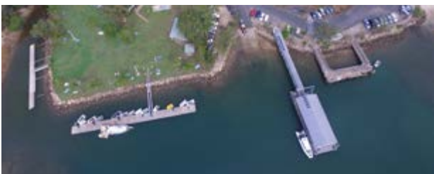
View of One Mile Ferry Terminal
