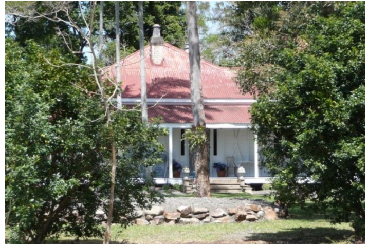
Birkdale House, Birkdale (RCC, 2012).
