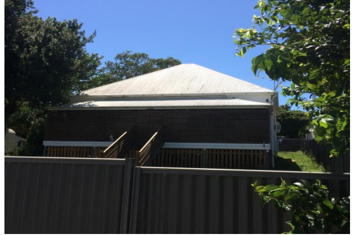
Residence, 14 Bingle Road, Dunwich (AHS, 2016).
