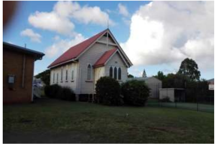
Former Methodist Church, Cleveland (AHS, 2017)
