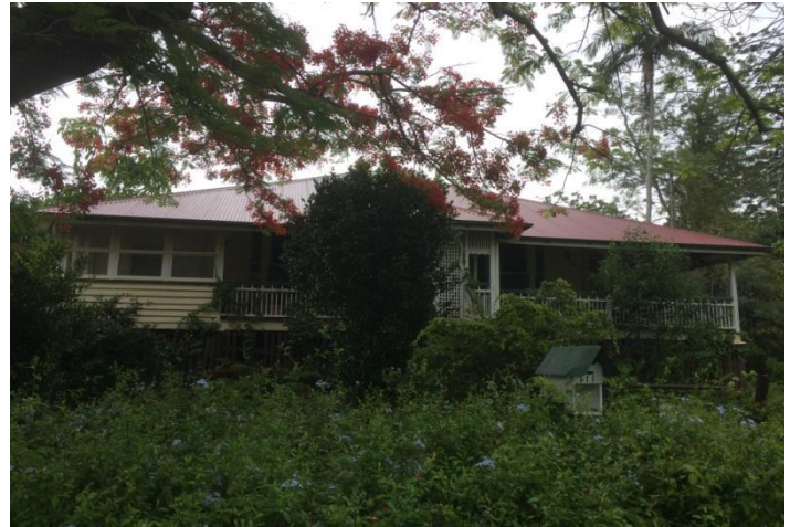
Residence, 111 The Esplanade, Redland Bay (AHS, 2016).
