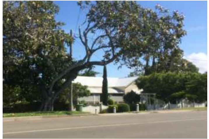
Residence, 19 North Street, Cleveland (AHS, 2017).
