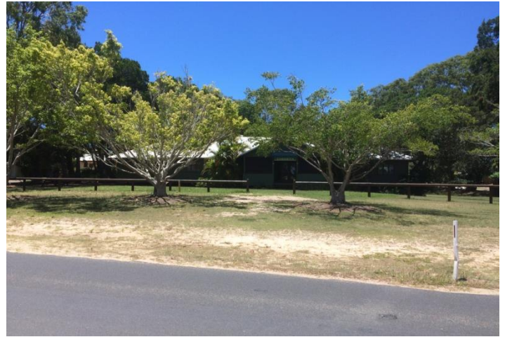
Residence, 2 Ballow Street, Amity Point (AHS, 2016).
