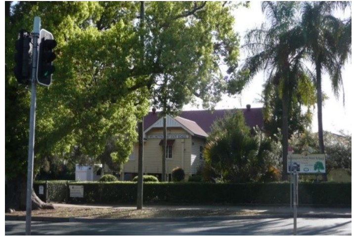
Wellington Point State School, Wellington Point (AHS, 2016).
