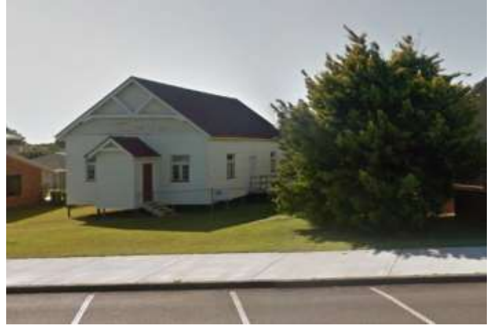
Methodist Church Hall, Cleveland (AHS, 2017).
