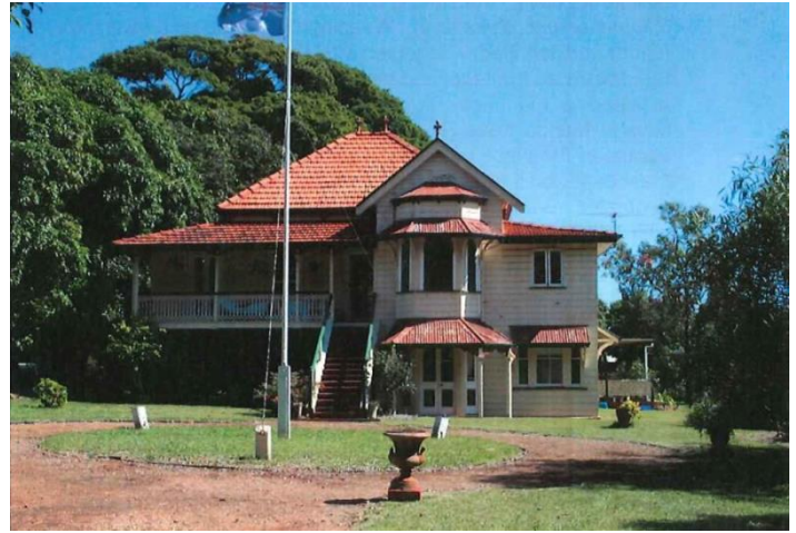
Somersby Grange, Birkdale (EHP, 2009).
