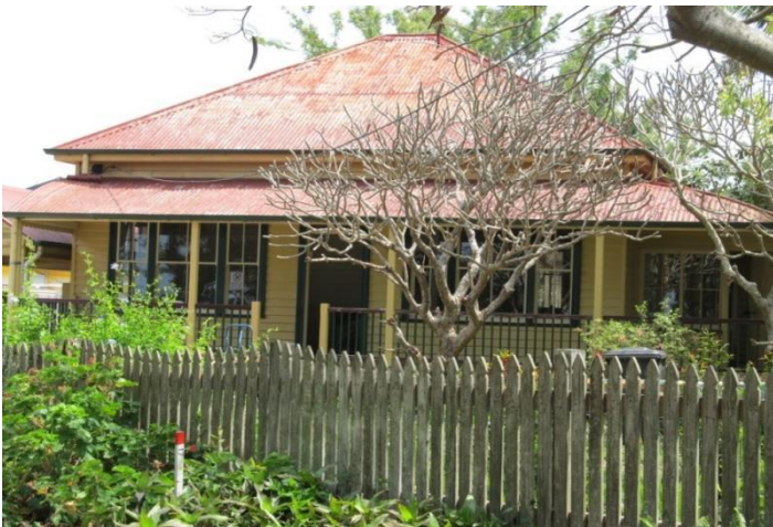
Residence, 17-18 The Esplanade, Wellington Point (RCC, 2012).
