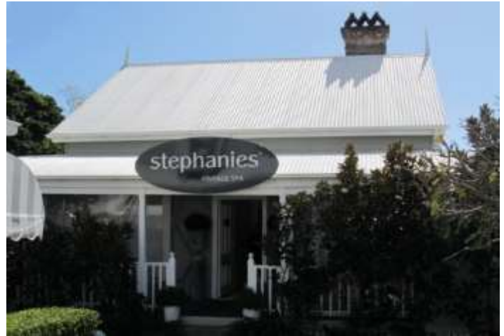
Residence, 200 Middle Street, Cleveland (RPS, 2012).
