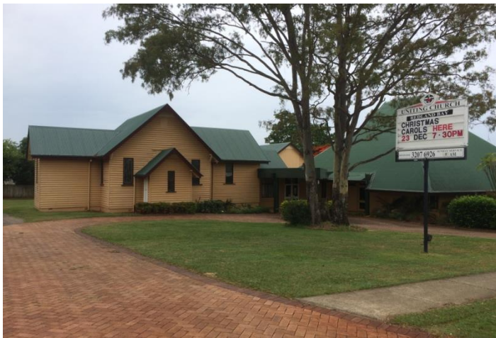
Former Methodist Church, Redland Bay (AHS, 2016).
