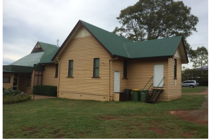
Former Methodist Church, Redland Bay (AHS, 2016).
