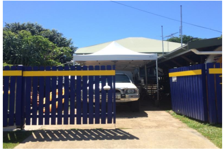
Residence, 18 Bingle Road, Dunwich (AHS, 2016).
