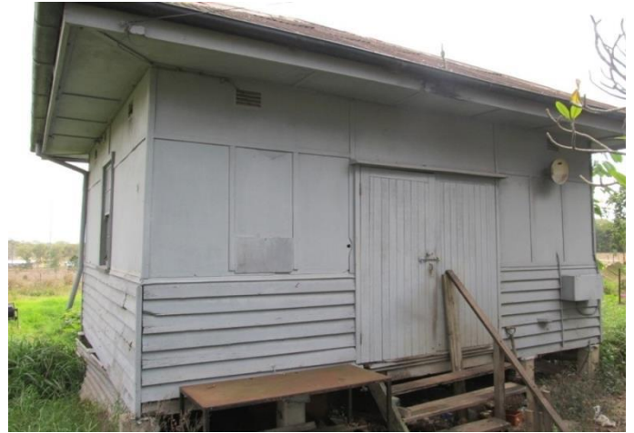
Small Hut on Old Cleveland Road East (AHS, 2016).
