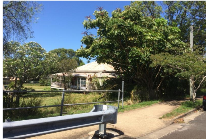
Residence, 3 Station Street/509 Main Road, Wellington Point (AHS, 2016).
