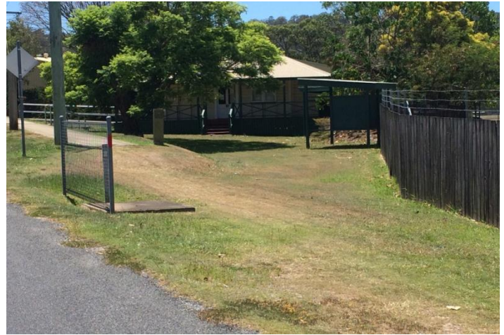
Residence, 8-22 Mallon Street, Dunwich (AHS, 2016).
