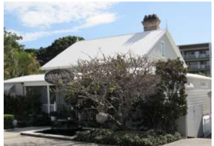
Residence, 200 Middle Street, Cleveland (RPS, 2012).
