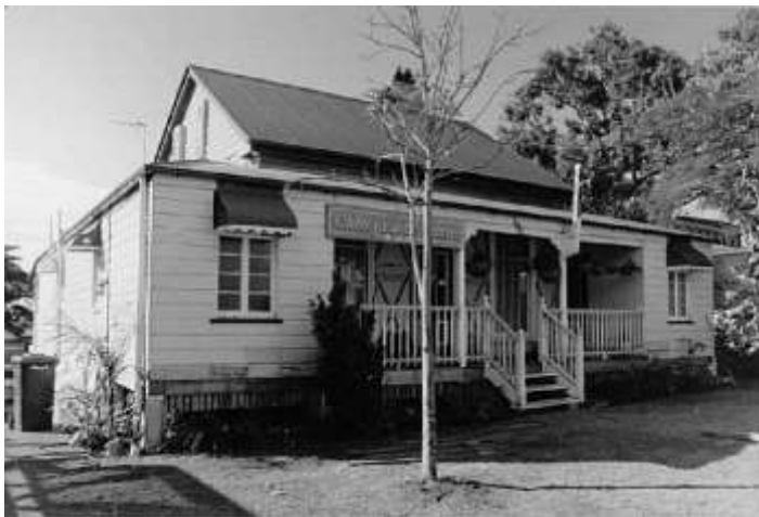
Residence, 200 Middle Street, Cleveland (RPS, 2012).
