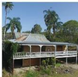
Historic Willards Farm, Birkdale (Cullen Cullen)
