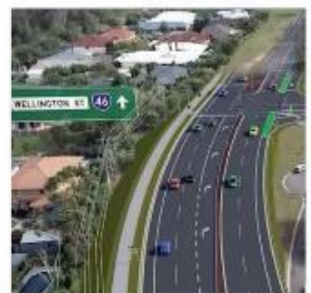
Wellington Street / Panorama Drive road upgrade program
