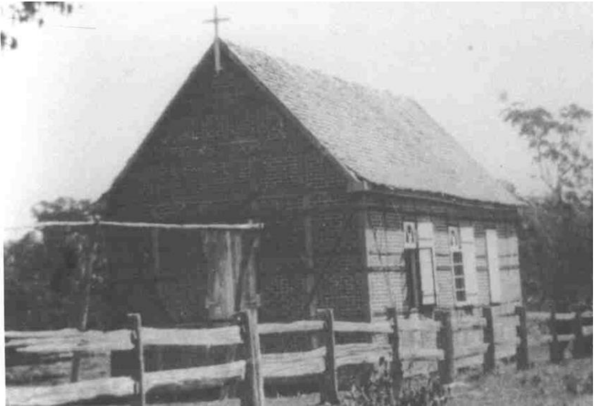
St Paul's Lutheran Church Mount Cotton, built in the Fachwerk style. Undated – however the shingle roof was replaced with an iron roof in the early 1920s, ahead of the church's 50 th anniversary. The cemetery grew behind it. HP01203
