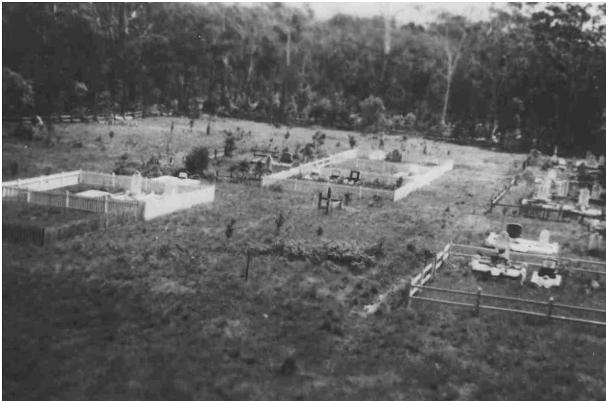
The Mount Cotton Cemetery at the corner of Wuduru and Mount Cotton Roads (near German Church Road) was photographed from the roof of the old church shortly before the building collapsed, 1951 HP01165
