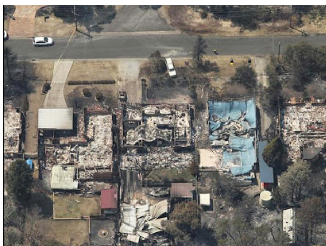
News Limited photograph of buildings in Winmalee, NSW that have succumbed to ember attack from the Blue Mountains, NSW fires in 2014. The unburnt condition of the vegetation around the buildings is evidence of ember attack on unprotected and probably undefended buildings.
