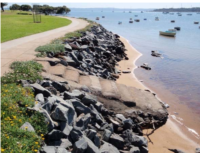
Figure 2 - Existing Stairs at 38 Orana Esplanade
