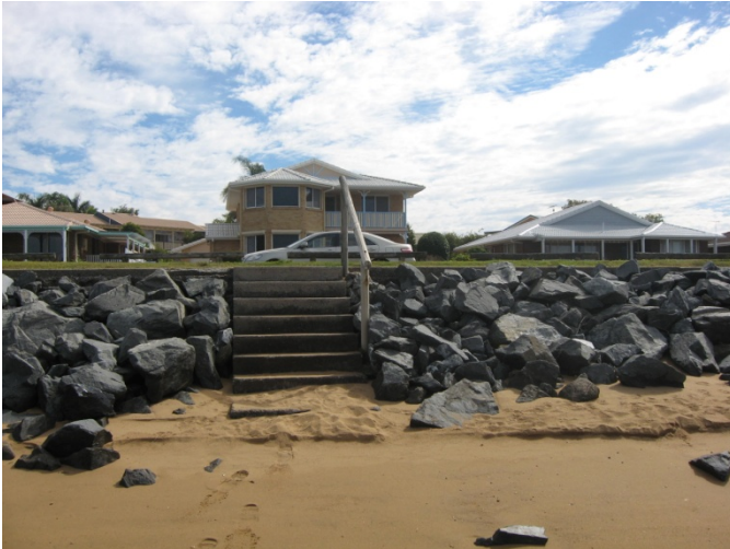
Figure 1 - Existing Stairs at 24 Orana Esplanade
